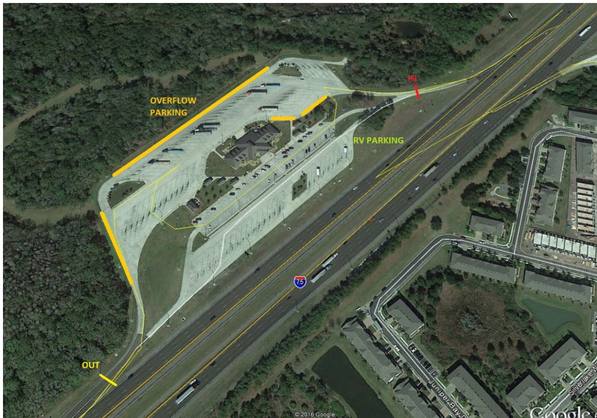
FIGURE 4 SOUTHBOUND I-75 PASCO REST AREA OVERFLOW PARKING
