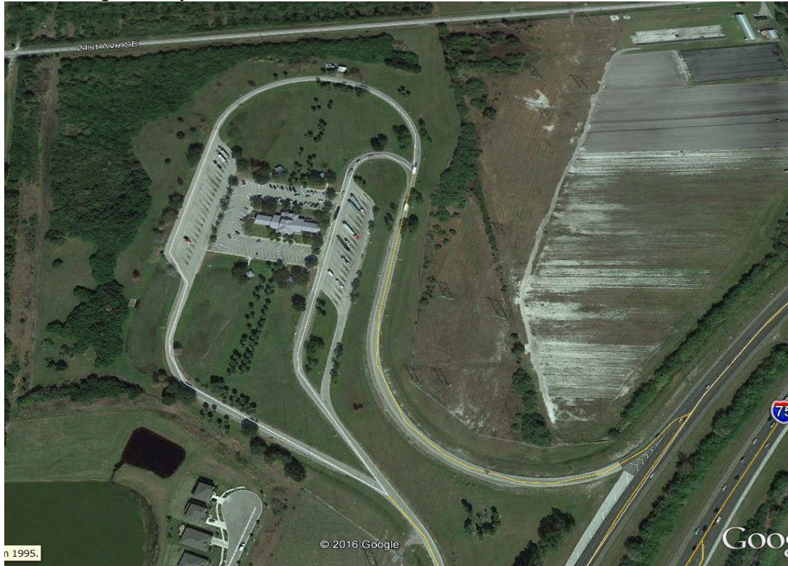
Hillsborough County I-75 Rest Area SB
