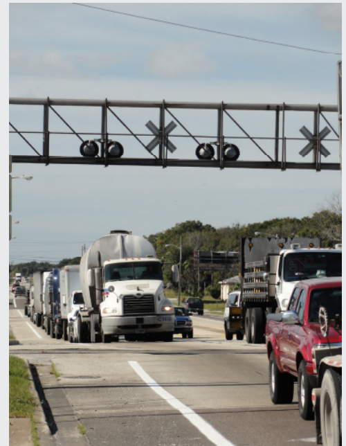
At-grade railroad crossings present design concerns for all travelers, with special operational concerns for goods movement.
