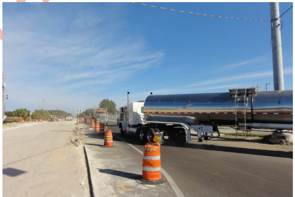
Encroachment during maintenance of traffic can be managed by a variety of active or passive control devices.
