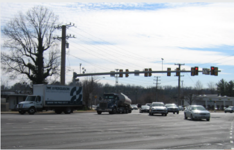
Multiple exclusive right turn lanes are particularly challenging for pedestrians unless right-turns on red are prohibited.
