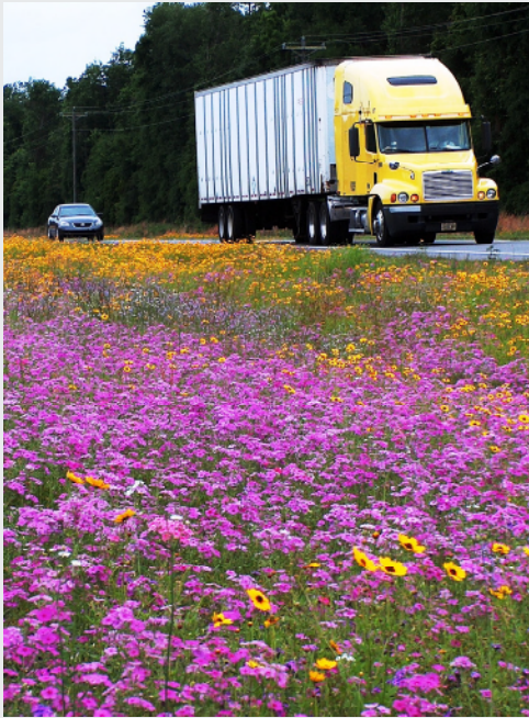
Effective landscaping can reinforce the roadway context in all types of context areas.
