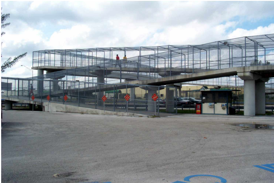
Photograph 2. Pedestrian Overpass Bridge.
