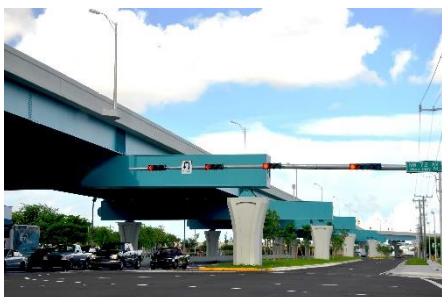
NW 25th Street Viaduct provides direct access between MIA and Doral warehousing District
