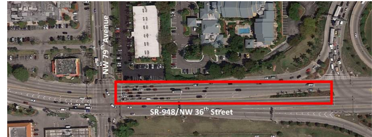
Figure 3.7: SR-948/NW 36th Street and NW 79th Avenue
