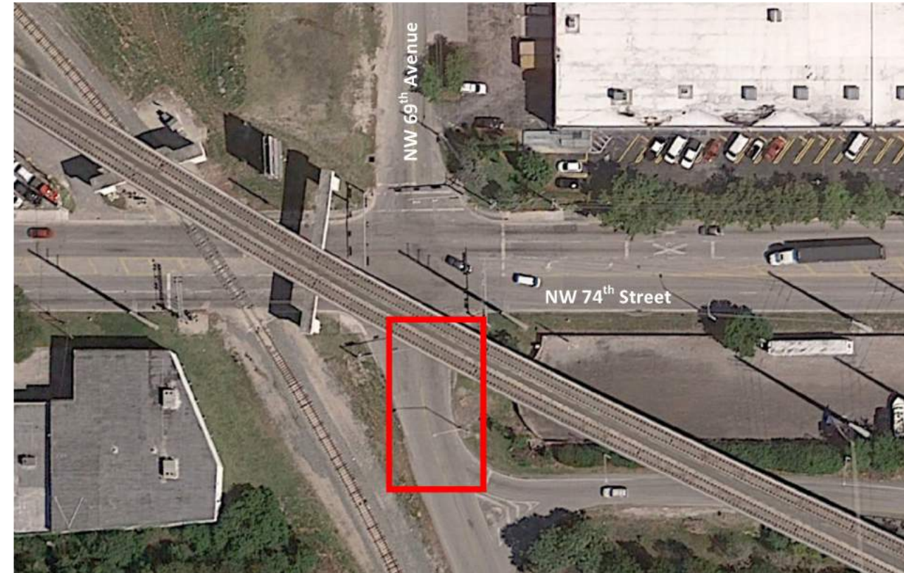
Figure 2.9: NW 74th Street at NW 69th Avenue
