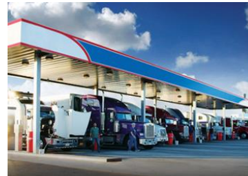
Figure 11: Diesel Fuel Station
