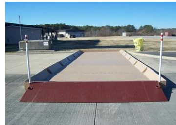
Figure 15: Leaky Load Cont.
