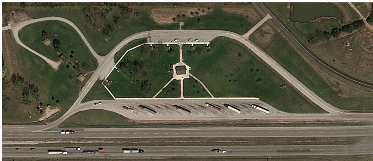
Figure 17a | Interstate 70 Rest Area in Danville, Missouri - Before Conversion
