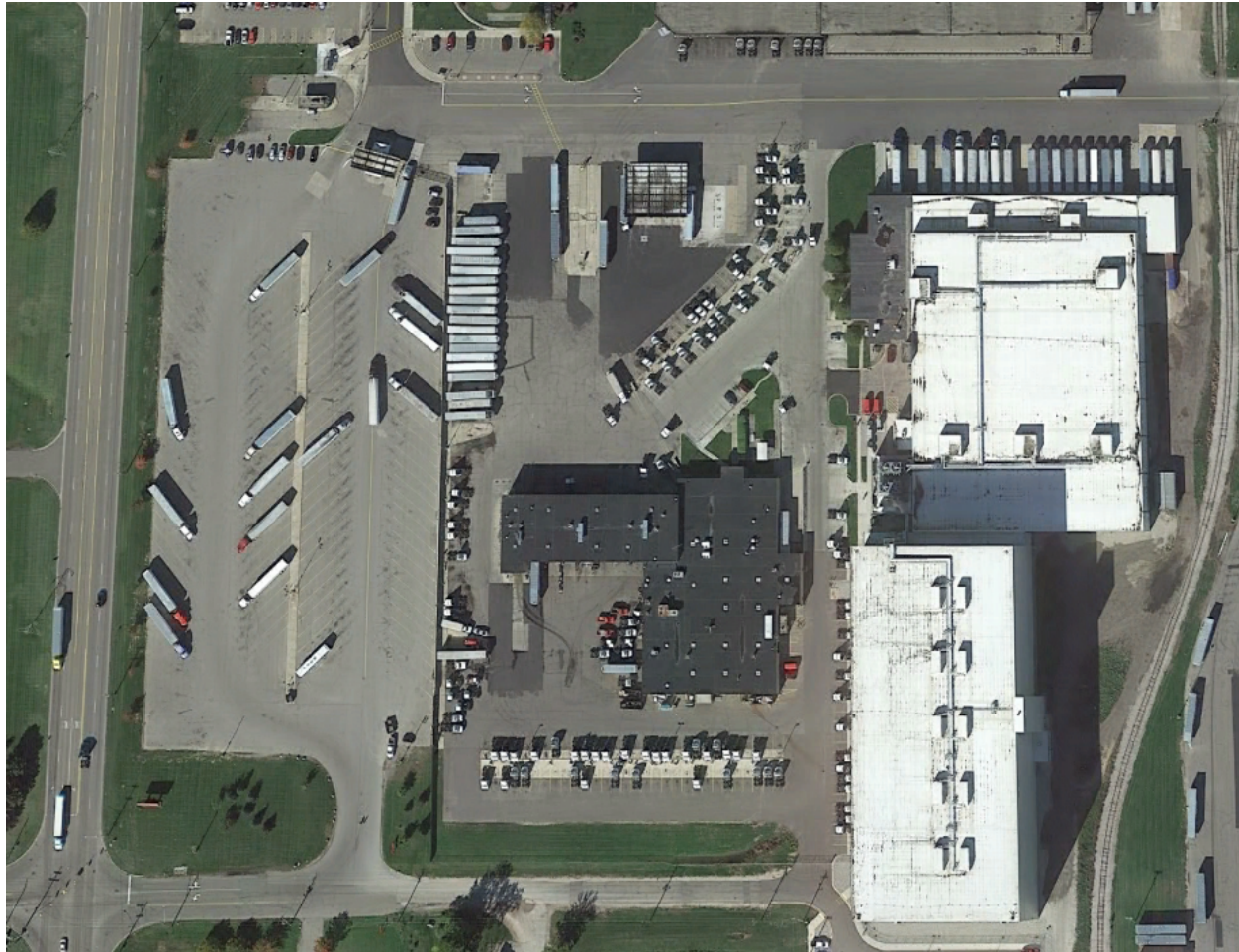
Figure 22 | Meijer Grocery Stores Distribution Center in Lansing, MI
