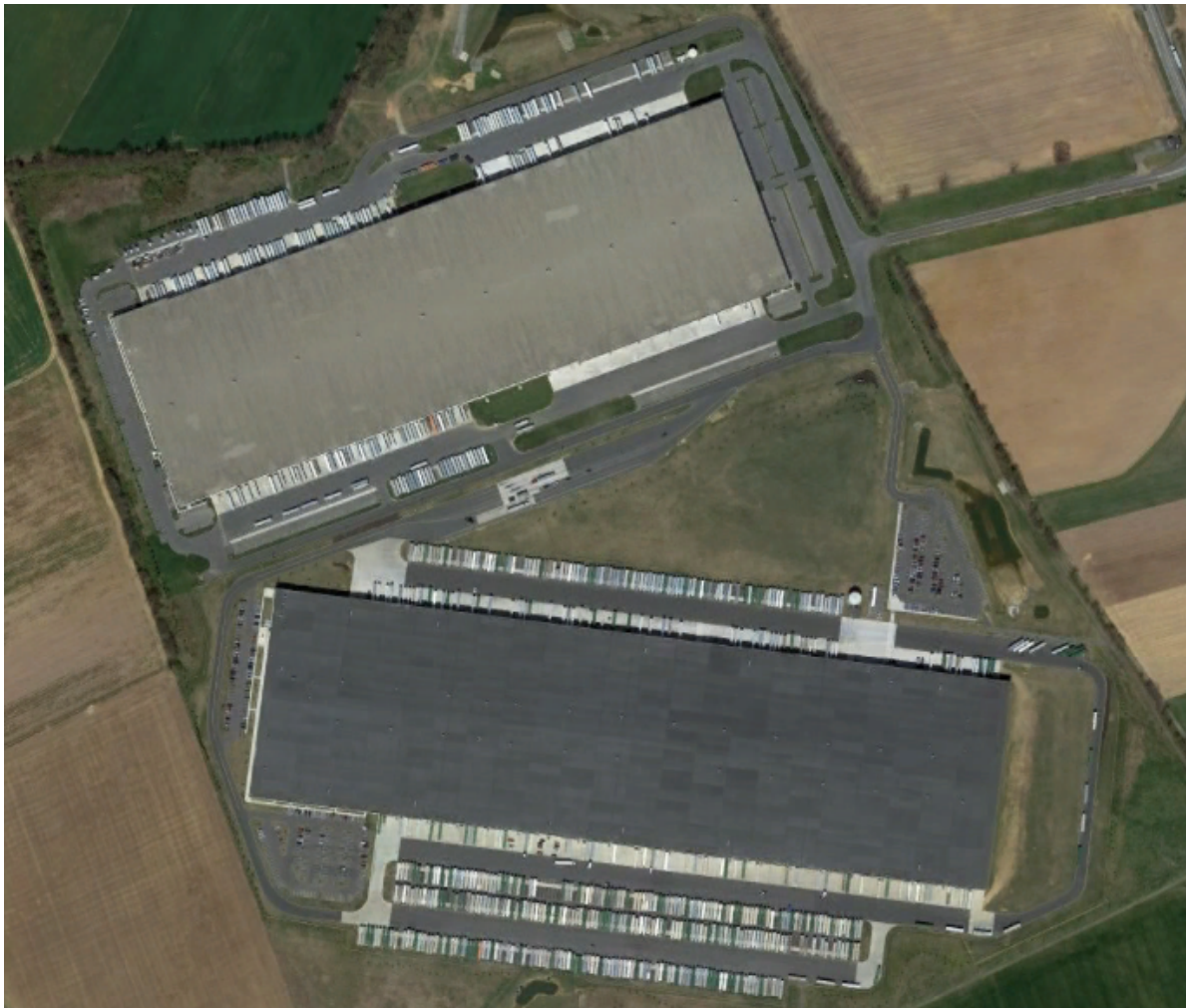
Figure 23 | Unilever Distribution Center in Newville, PA
