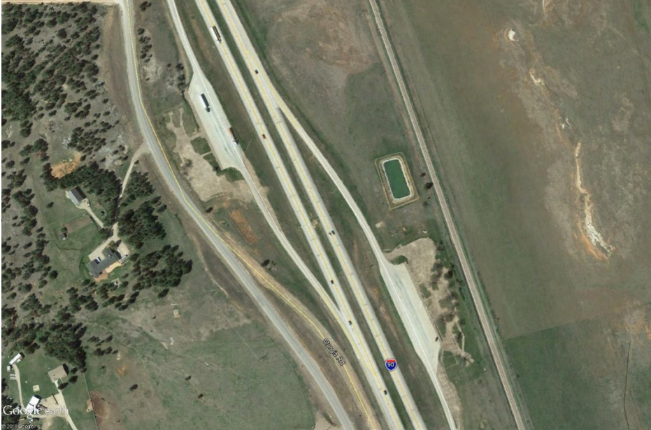
Figure 18 | Truck-only parking facility in South Dakota
