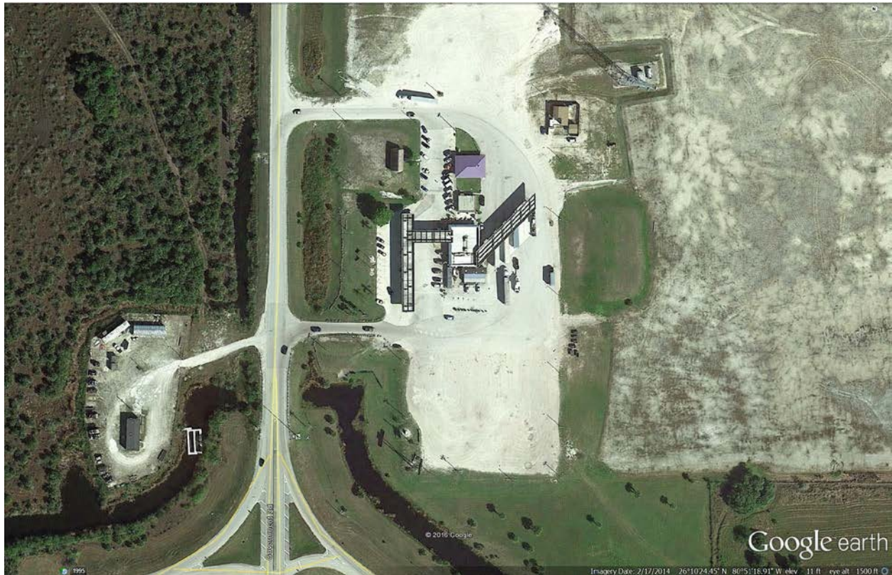
Figure A.48 Google Earth Aerial of Miccosukee Service Plaza
