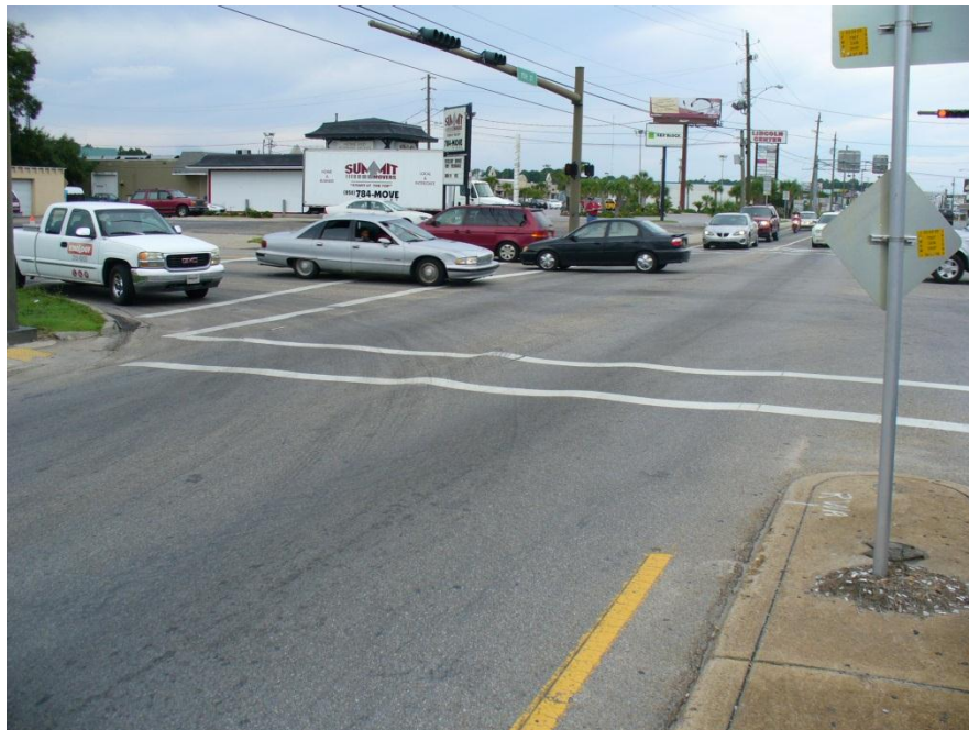
Photo 3 Rutting throughout the US 98/Jenks Avenue intersection forms a checker pattern, creating a rough intersection for travel in all directions.
