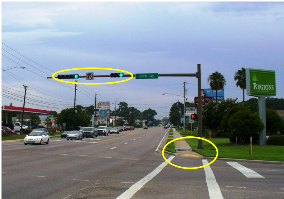
Photo 2 Eastbound traffic signals with no back plates. Infrastructure outside sidewalks away from road and corners.
