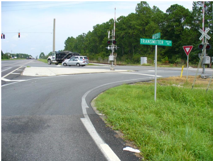
Photo 2 Railroad crossing gates on right-turn lane. Gate mounted on the raised island is for the southbound through traffic.
