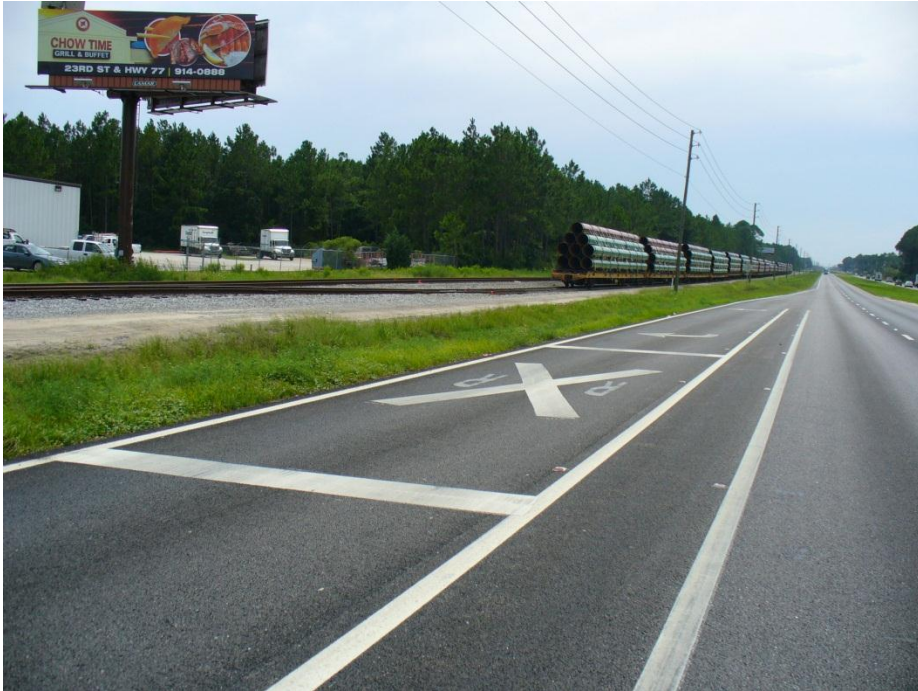
Photo 1 Right-turn only lane on US 231 with railroad warning pavement markings.
