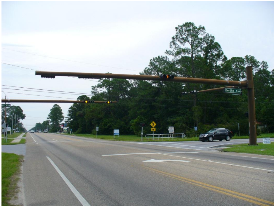
Photo 2 SR 22 intersection typical section. Includes signal-protected left-turn lane and mast arm mounted on traffic signals.
