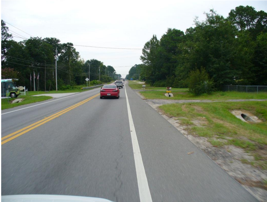
Photo 1 SR 22 typical section, two-lane with 5-foot paved shoulders and open drainage.
