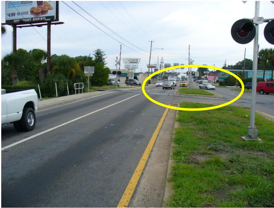
Photo 1A Railroad crossing on US 98, west of Harrison Avenue. Note the unsignaled left-turn lane to US 231)
