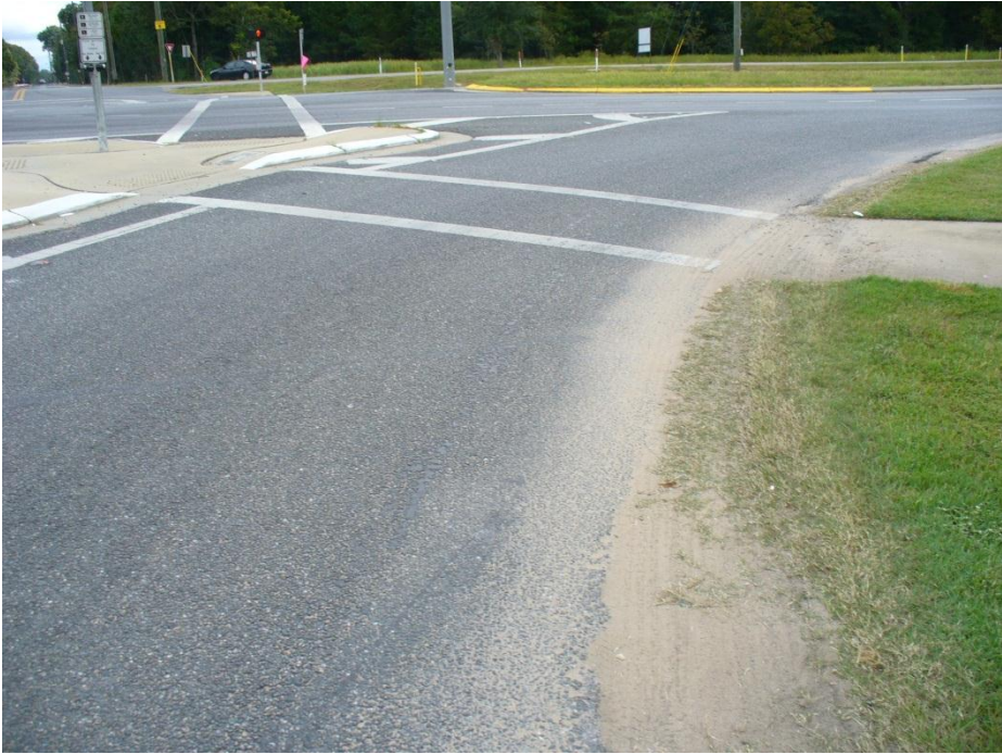
Photo 9 Channelized right-turn lane and raised concrete island at the northeast corner of Airport Road
