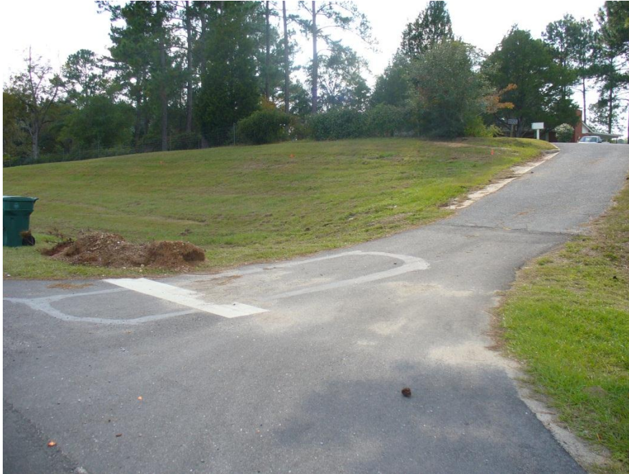
Photo 1 Signalized private driveway opposite Business Park Road (note the loop detector and stop bar)
