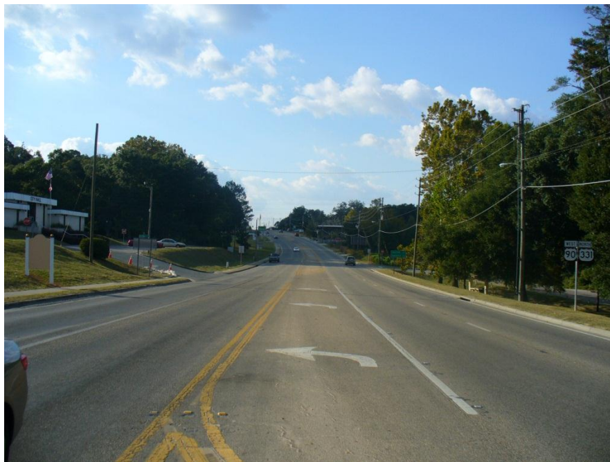
Photo 2 Five-lane typical section on US 90/US 331
