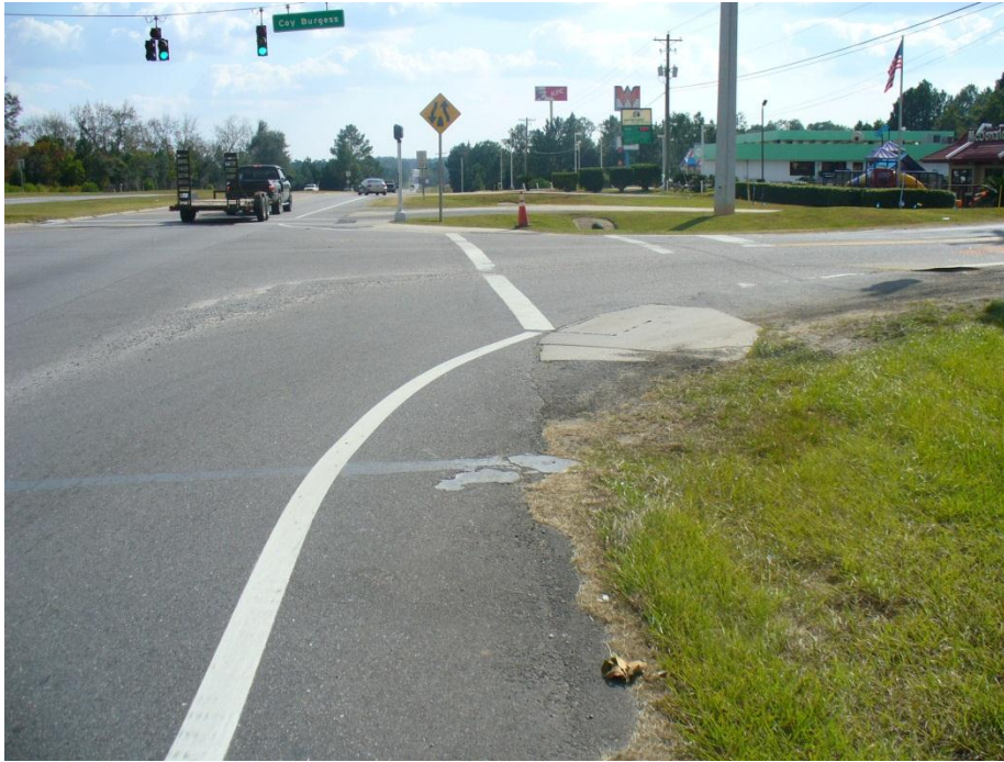
Photo 5 New traffic signals and pedestrian features at Coy Burgess Road (also note off-tracking damage at the northbound corner)
