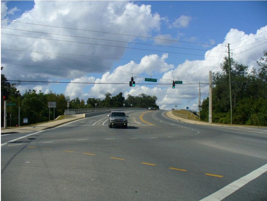
Photo 3 Approach to grade-separated railroad bridge west of Ward Basin Road
