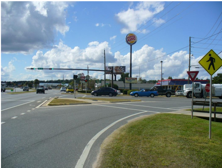
Photo 4 US 90 at SR 87 (Stewart Street) channelized right turn with grass island
