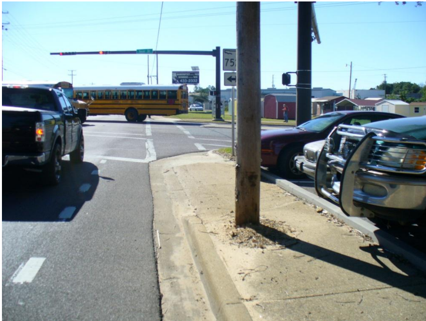
Photo 4 Poorly located utility pole is too close to the roadway. Location may also pose a safety issue for wheelchair-bound persons.
