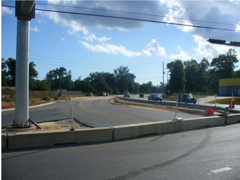
Photo 7 New construction at Avalon Boulevard
