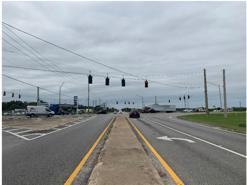
Intersection of US 27 and US 98
