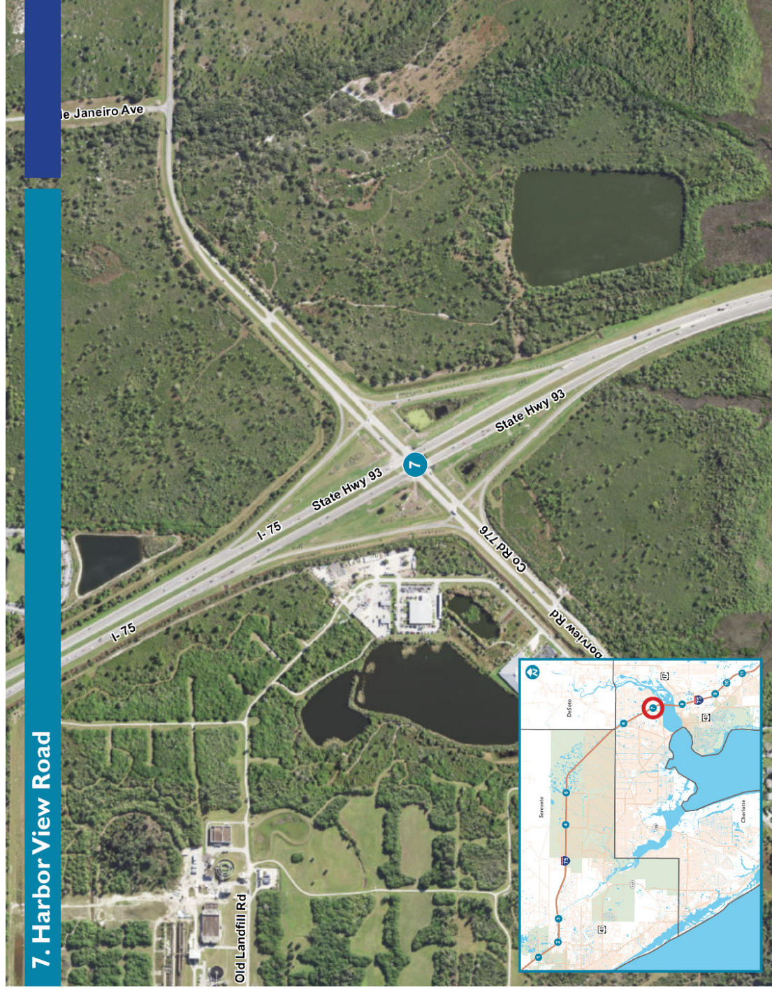
Figure 14: I-75 and Harbor View Road Interchange
