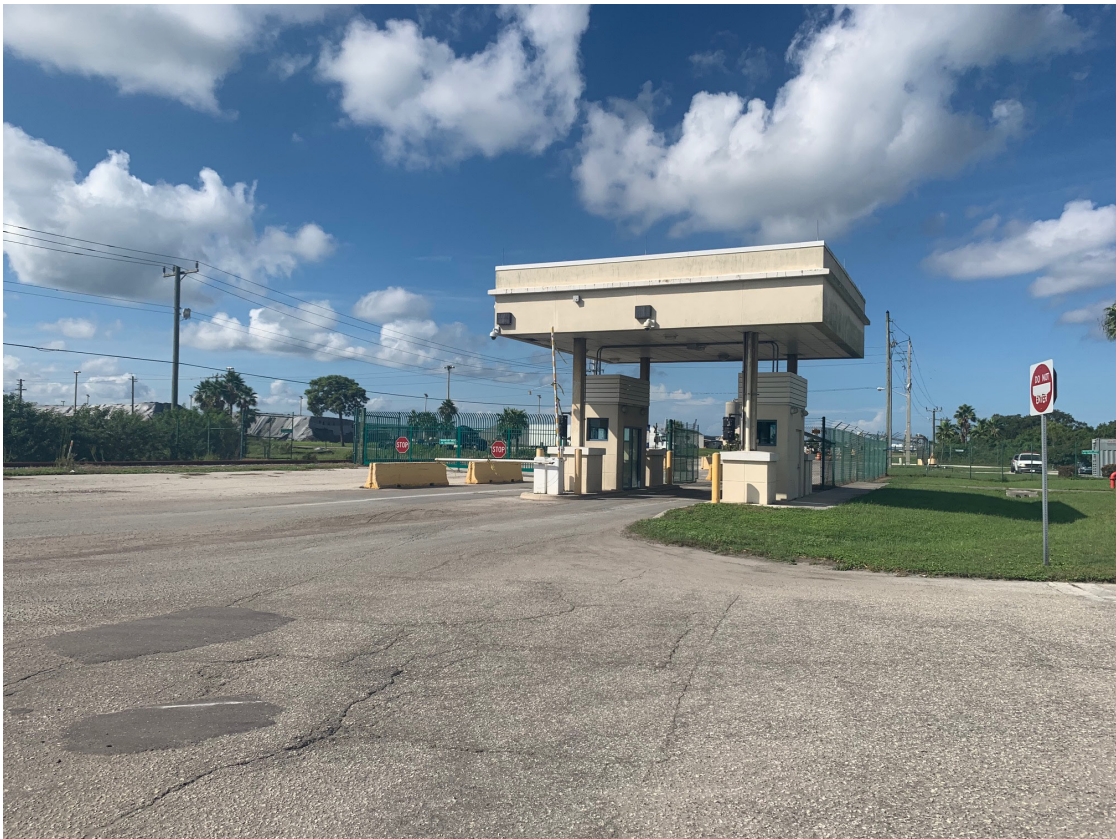
Figure 9: North Dock Street (West)
