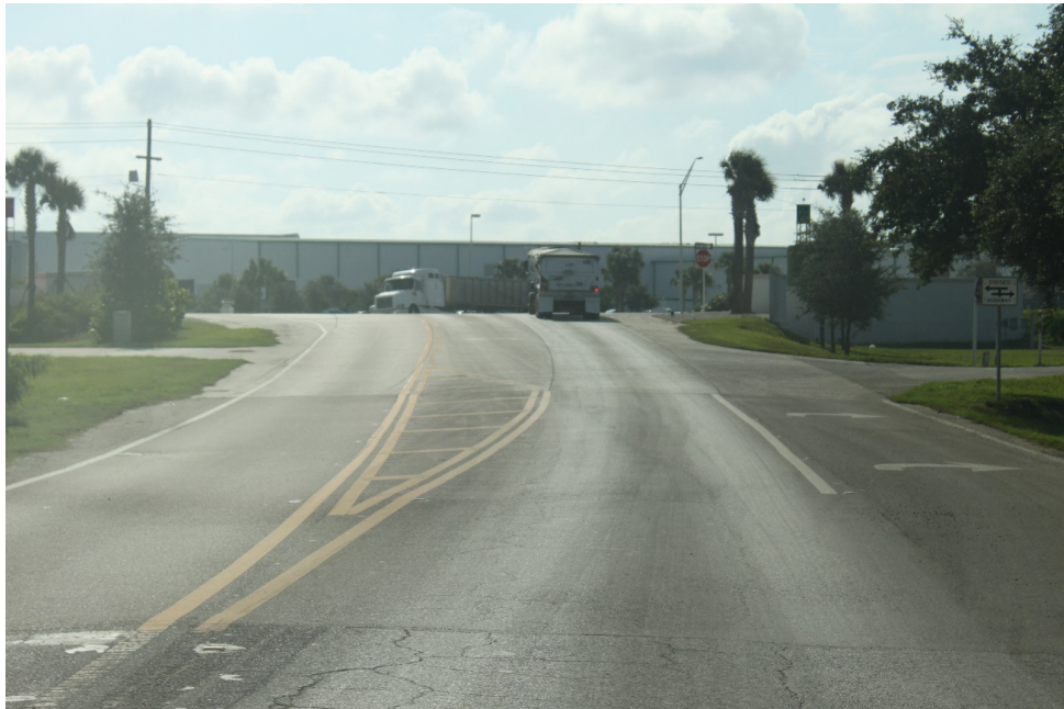
Figure 6: Intersection of US 41 and Piney Point Road
