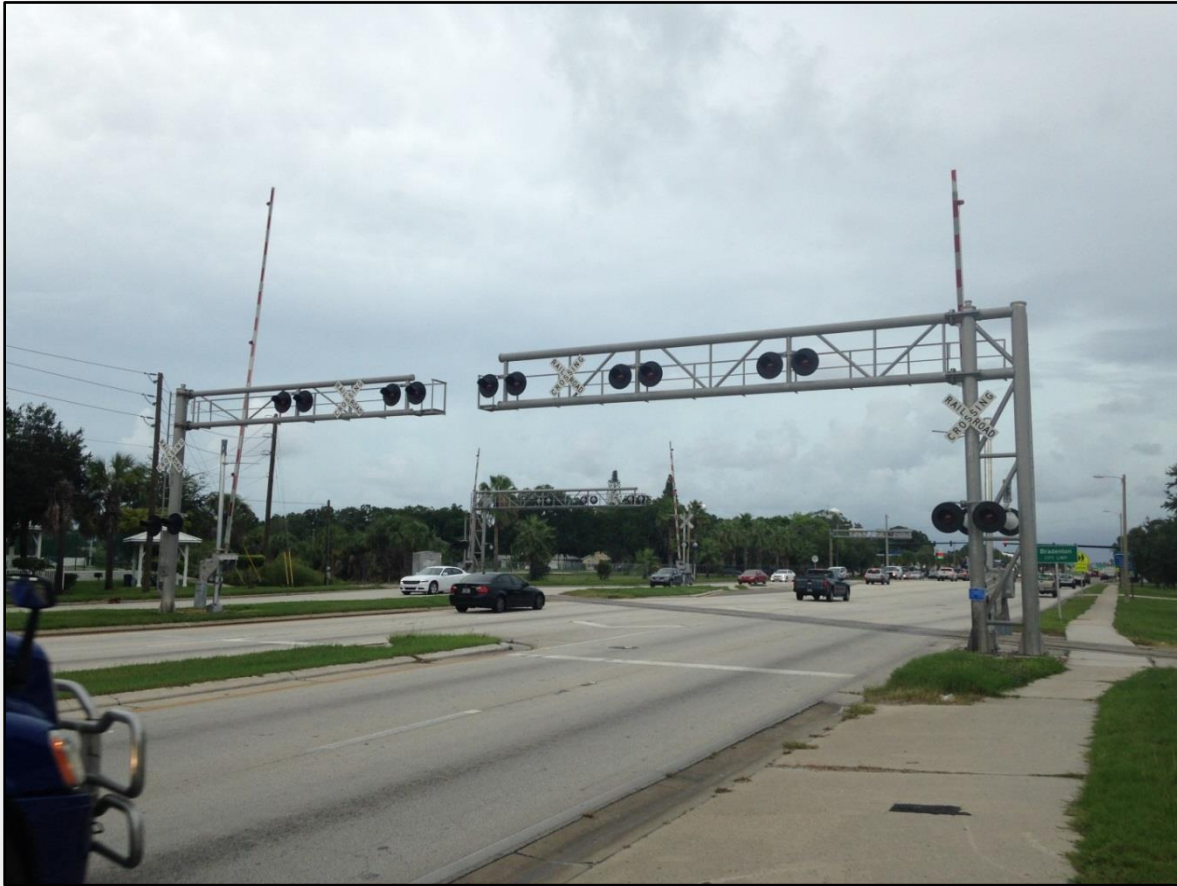
Figure 3-2: Site Visit: US-41/301 / SR-55/683 – Manatee County
