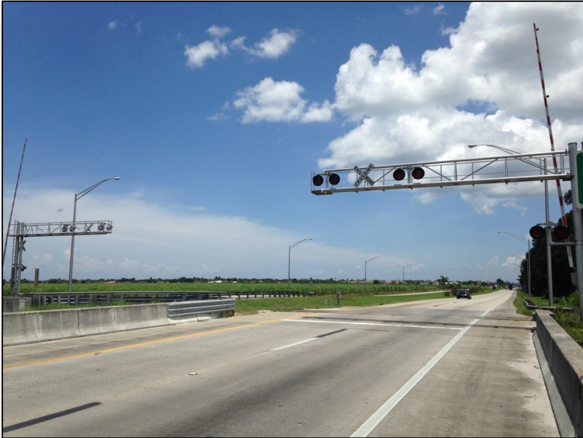
Figure 3-7: Site Visit: US-27/SR-80/SR25 – Hendry County
