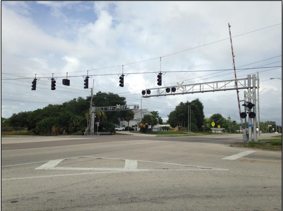
Figure 3-4: Site Visit: US-92/600 (Fish Hatchery Road) - Polk County
