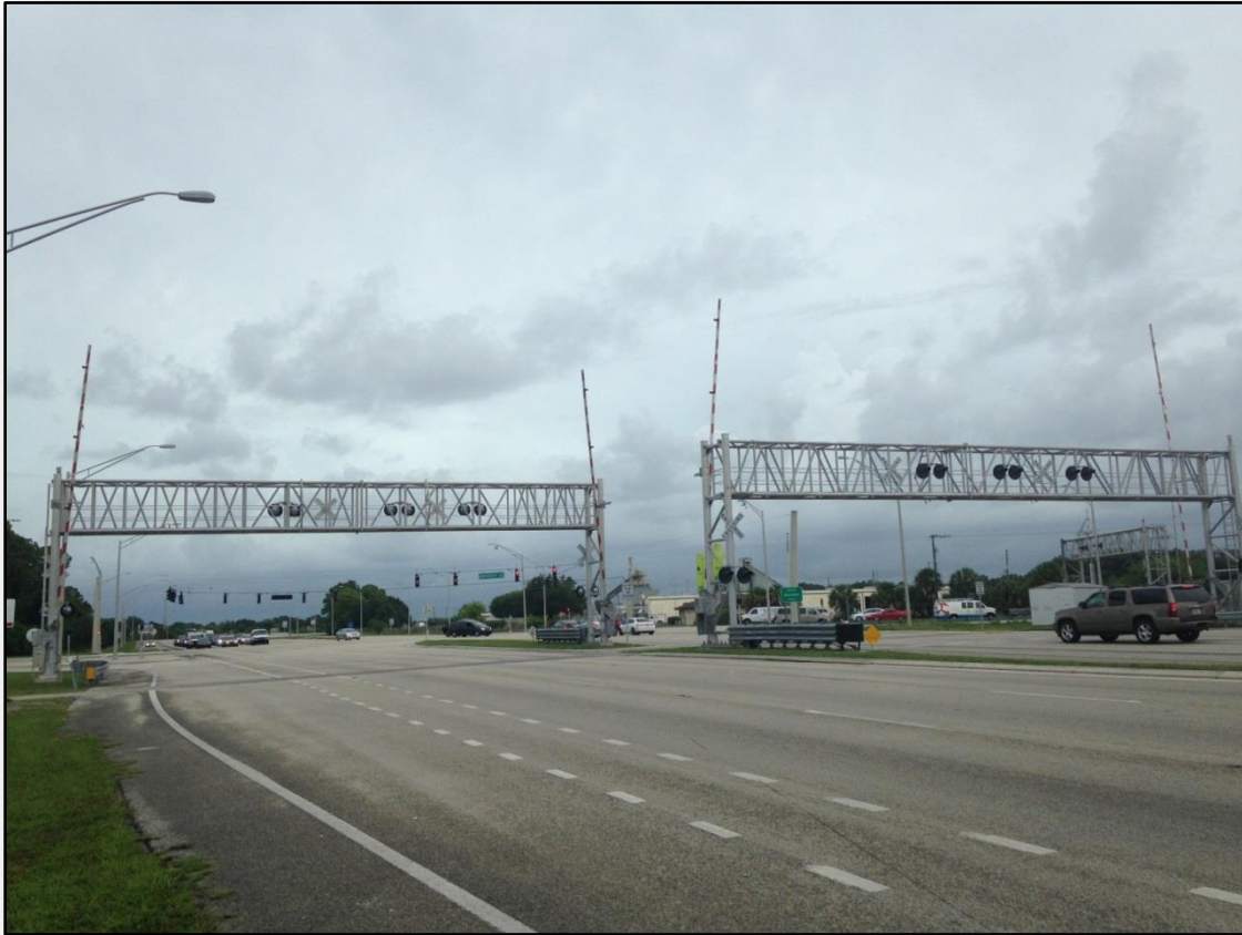
Figure 3-6: Site Visit: US-301/N Washington Boulevard – Sarasota County
