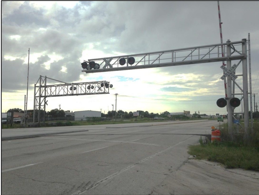
Figure 3-5: Site Visit: SR-60/Nichols Rd – Polk County
