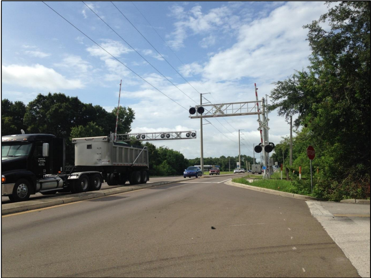
Figure 3-1: Site Visit: SR-659/Combee Road - Polk County
