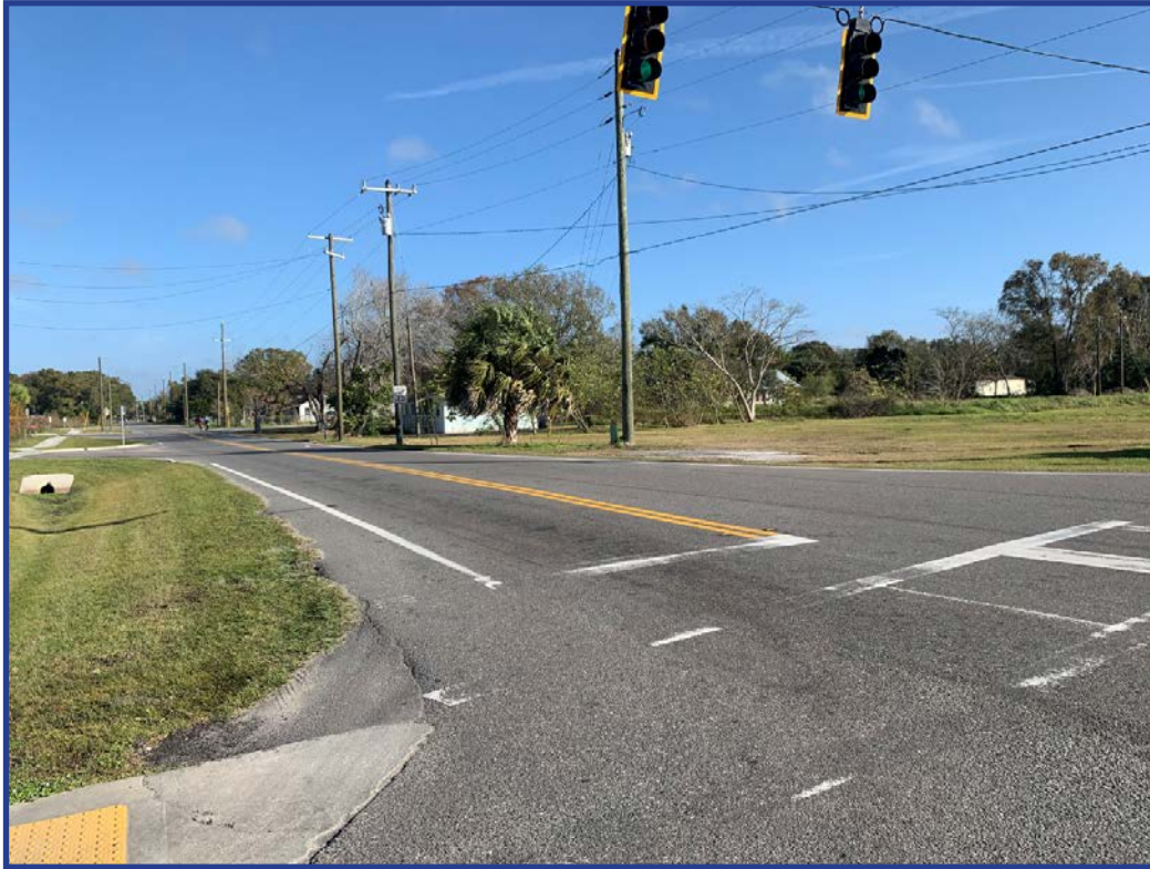
Figure 90: Looking North to old Bartow Lake Wales Road
