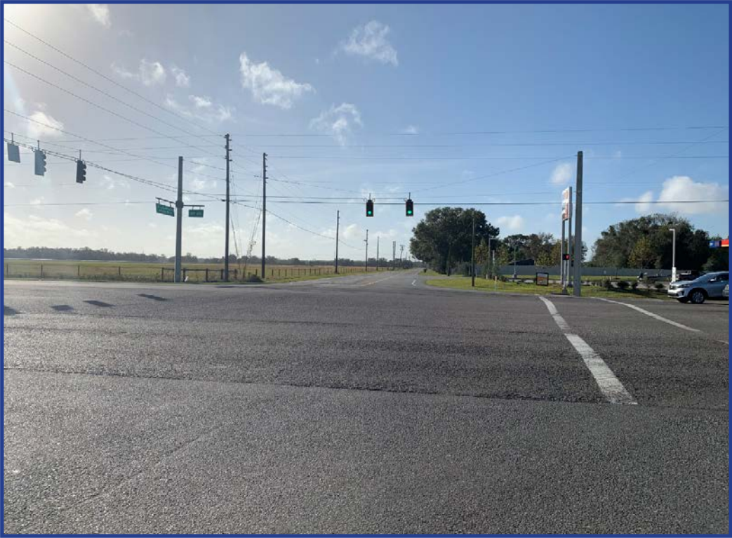
Figure 86: Looking South from SR 60
