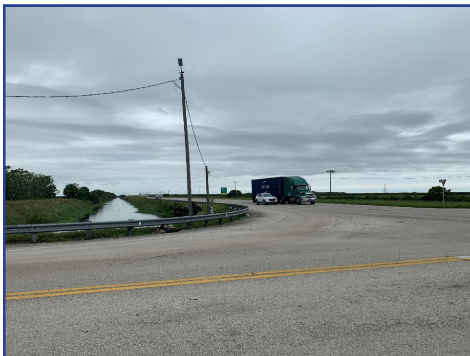
Figure 4: Flaghole Road Looking Northwest to US 27
