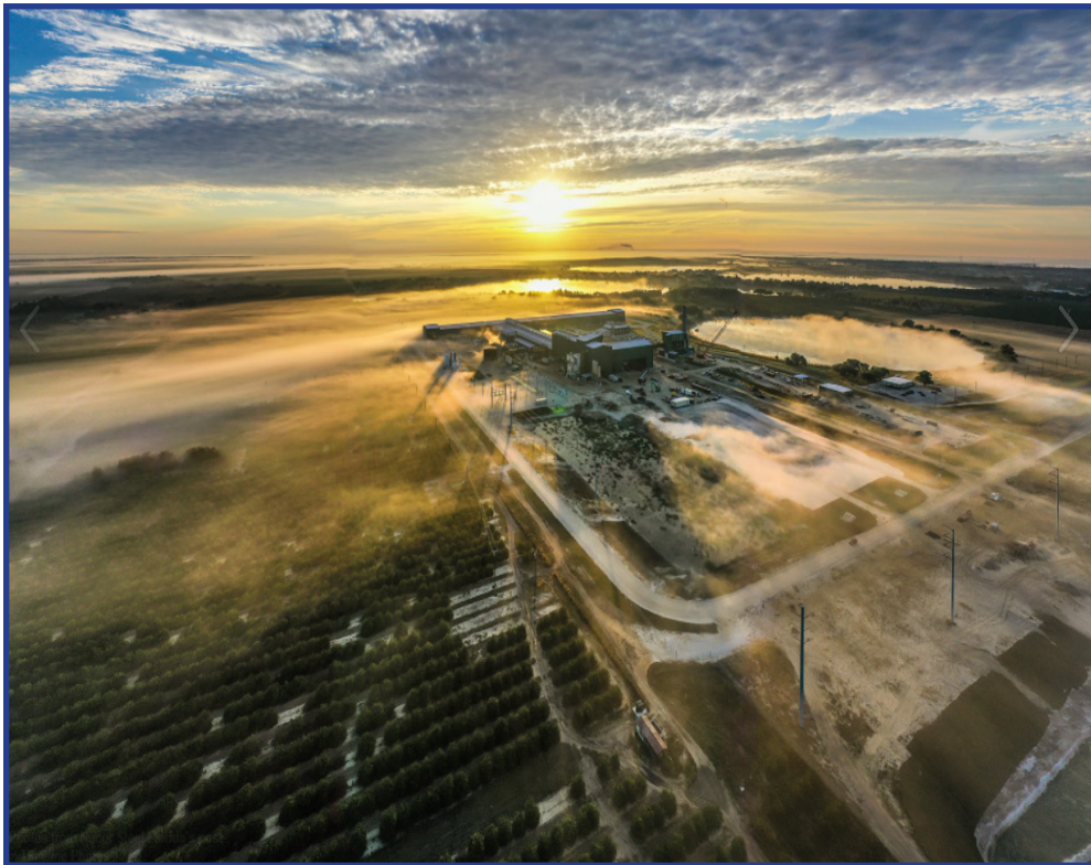
Figure 142: Nucor Steel Mill Aerial (Source: https://www.facebook.com/NucorFlorida/photos/ )
