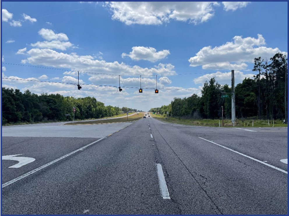
Figure 100: US 27 Looking South from US 17
