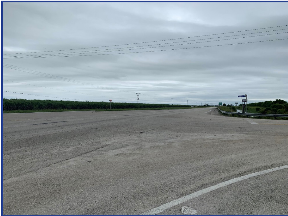
Figure 6: US 27 Looking East at US 27 from its Intersection with Flaghole Road
