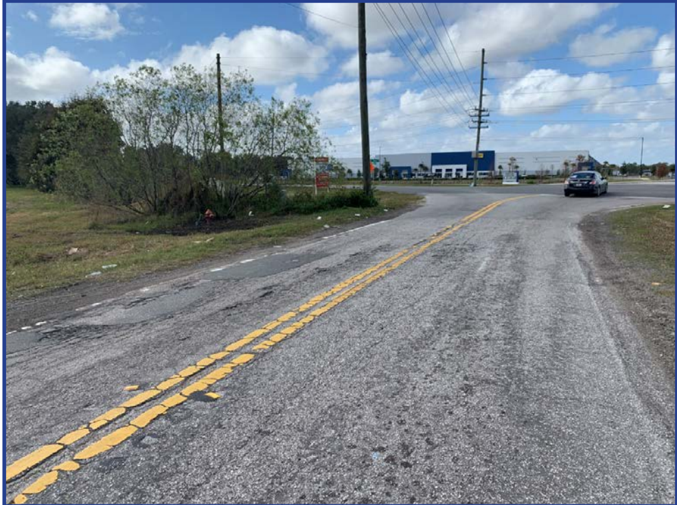
Figure 57: Road Conditions on Church Road Approaching the Intersection from the East
