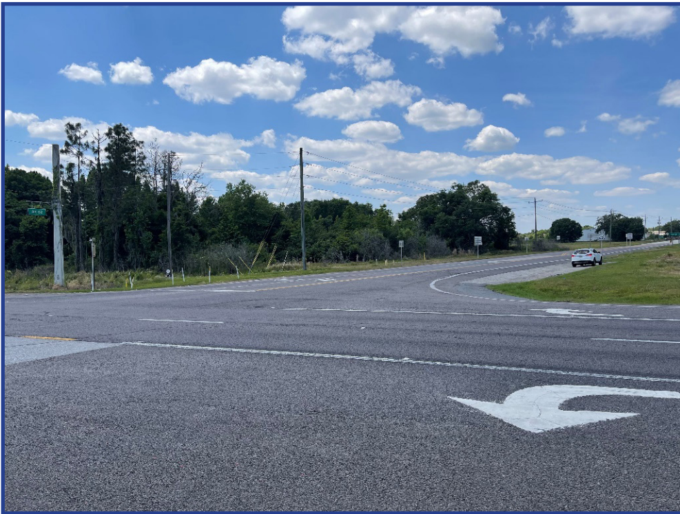
Figure 103: Looking at SR 62 from US 17
