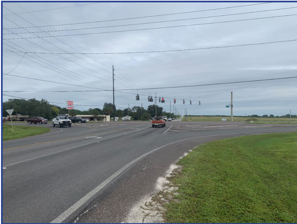
Figure 32: Looking East at the Intersection from CR 640
