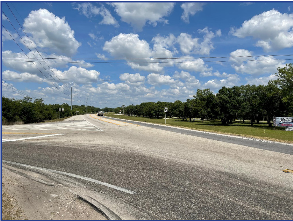
Figure 114: US 27 Looking Northwest on SR 70
