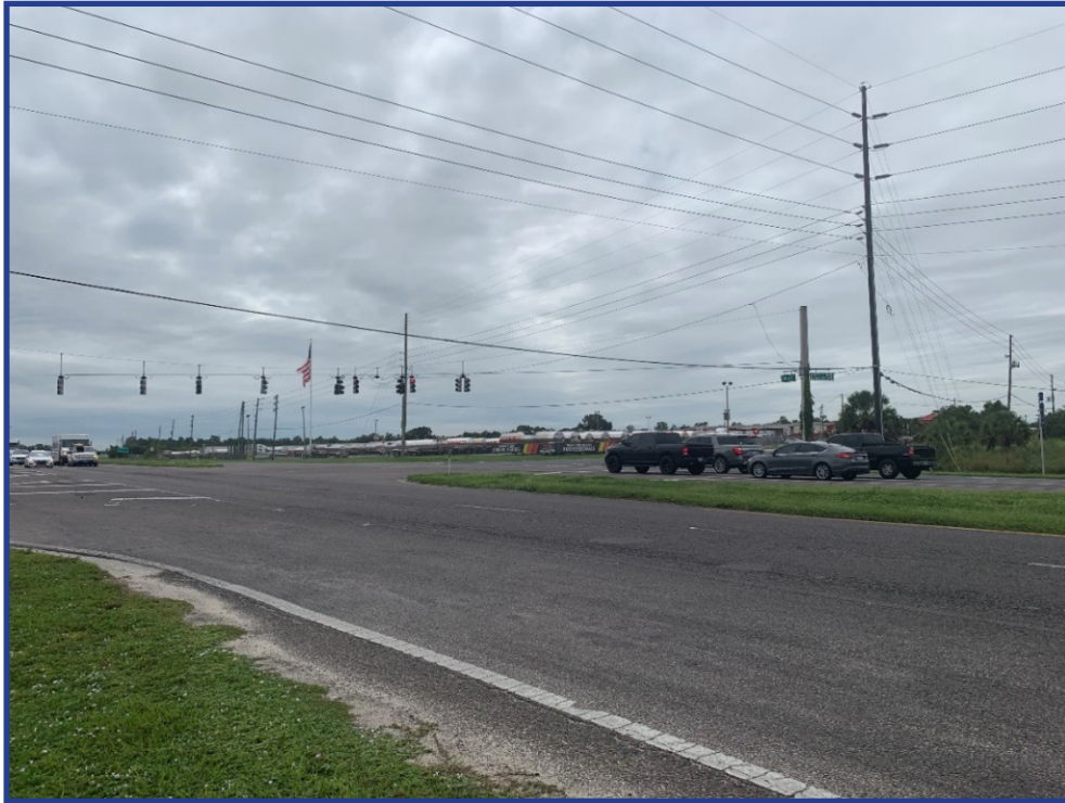
Figure 31: Looking Southwest from US 27
