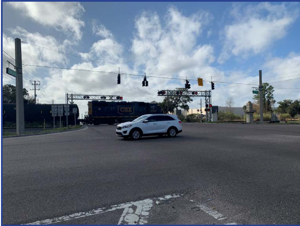
Figure 156: Looking South to At-Grade Crossing on US 92 from the Northeast
