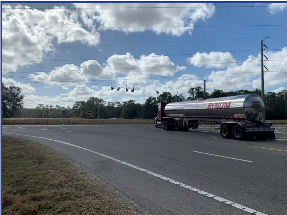
Figure 42: SR 471 Looking South to US 98
