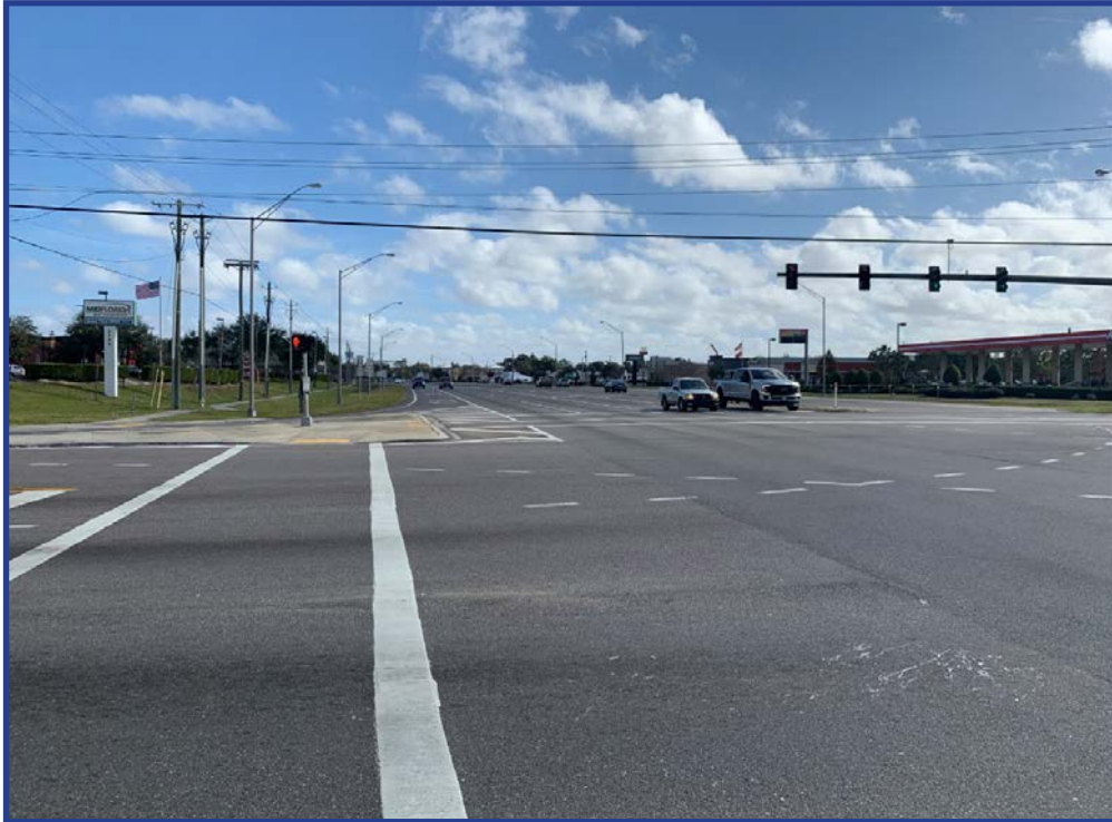
Figure 69: Looking East to US 92 from SR 559 (Berkley Road)
