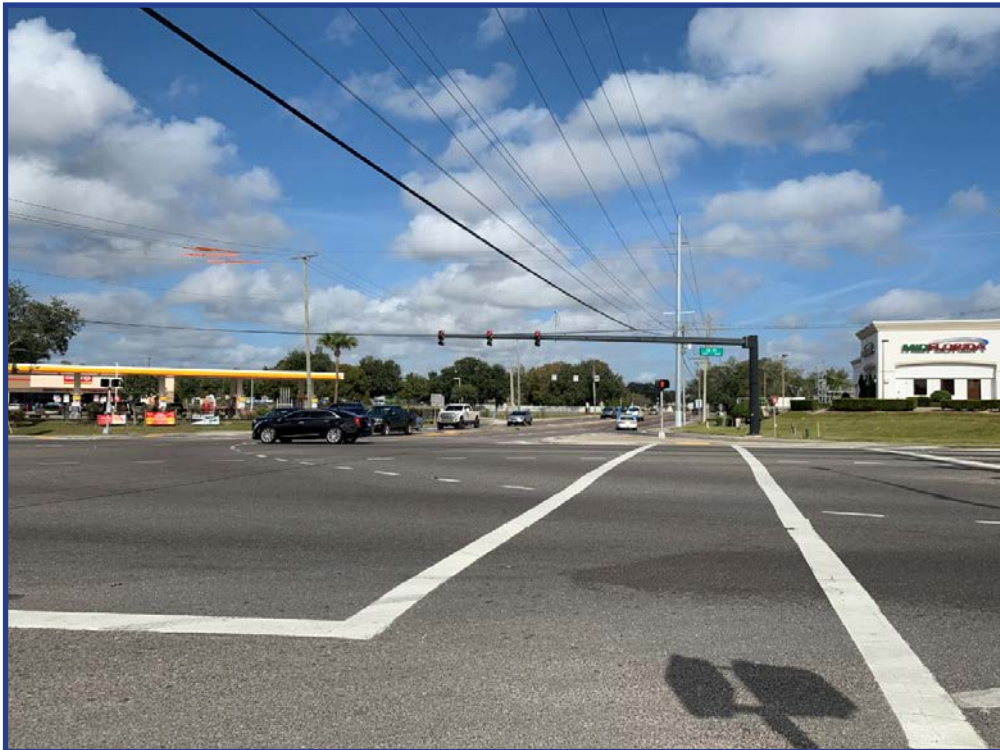
Figure 74: Looking North to SR 559 (Berkley Road) from Neptune Road
