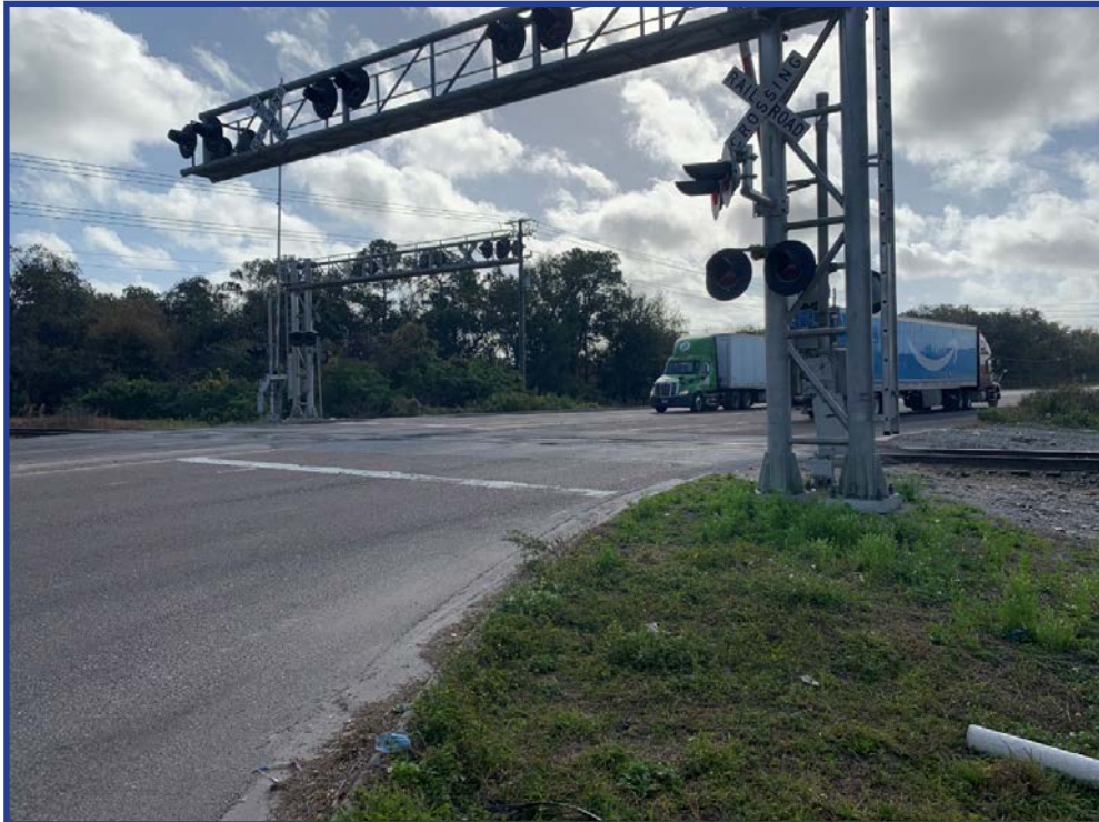
Figure 155: At-Grade Rail Crossing Located on US 92 - South of Intersection
