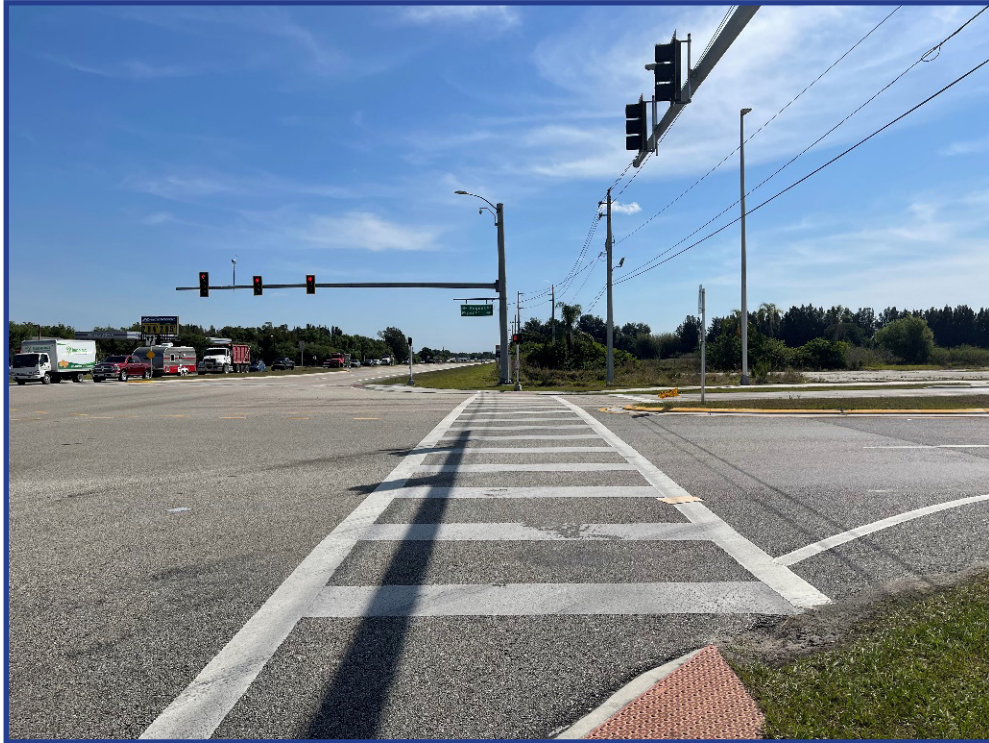
Figure 126: US 27 Looking East from US 17
