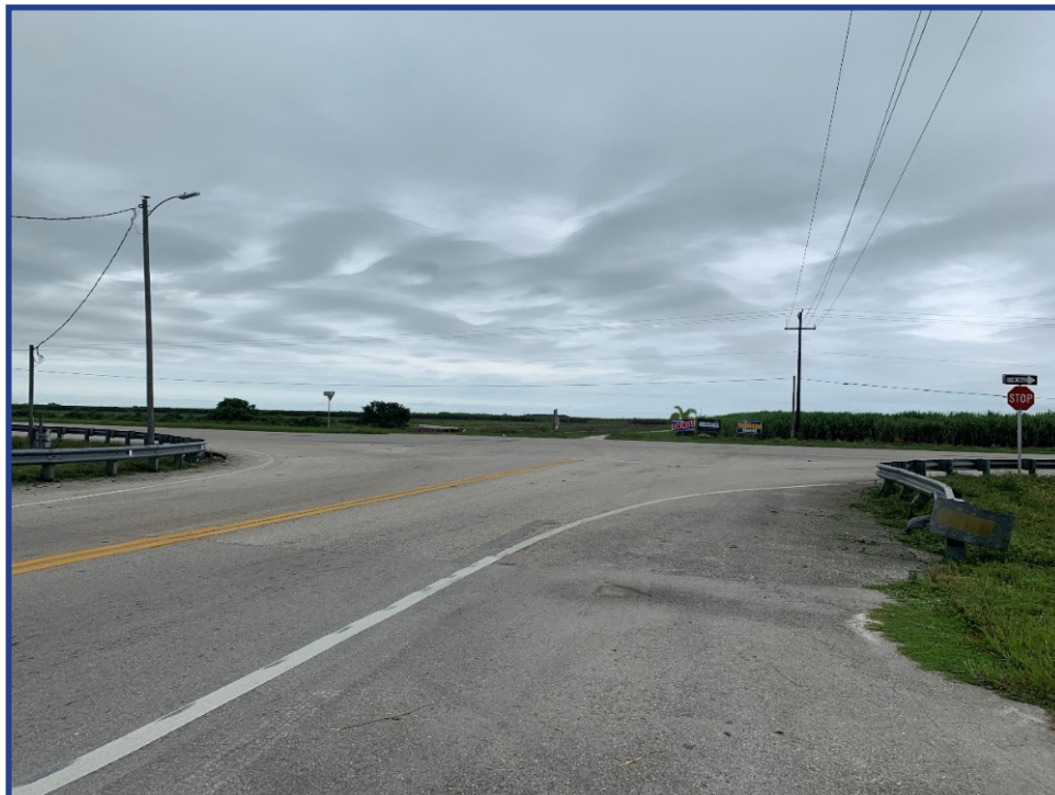
Figure 3: Flaghole Road Looking North to US 27
