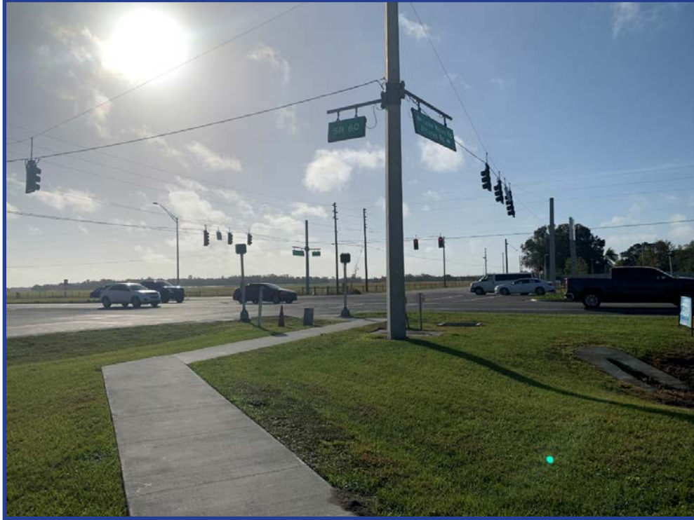
Figure 82: Intersection of SR 60 and Alturas Road / Old Bartow Lake Wales Road from the Northwest
