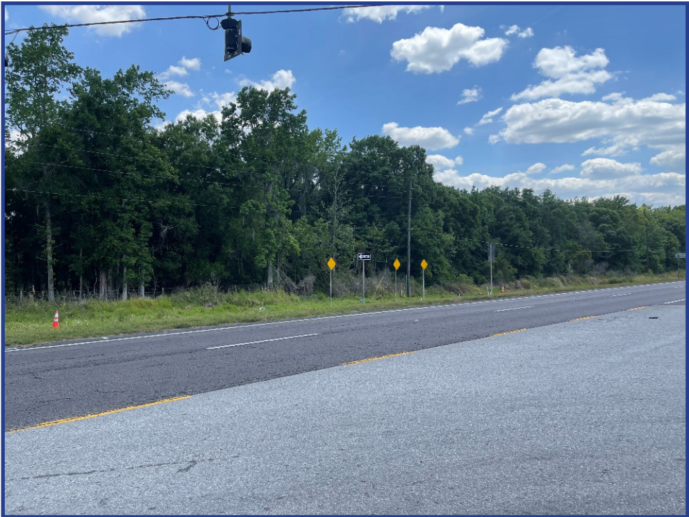
Figure 101 :View of the East Side of the Intersection
