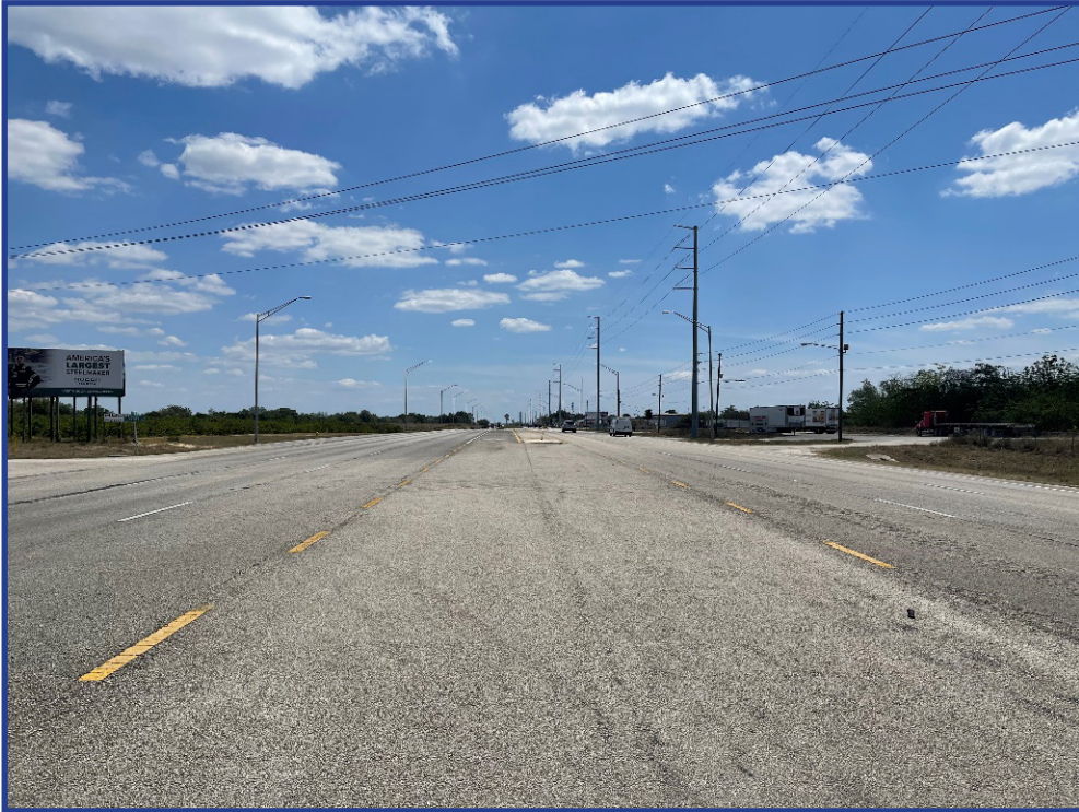
Figure 139: Looking Southeast on US 27
