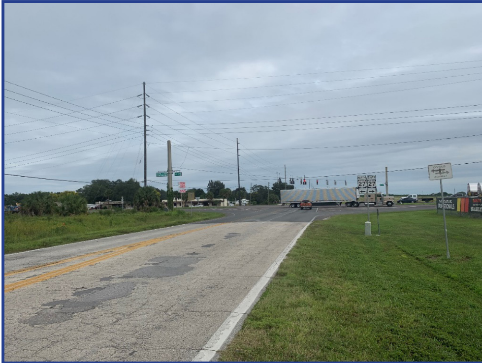
Figure 33: Roadway Conditions Approaching the Intersection from the West on CR 640
