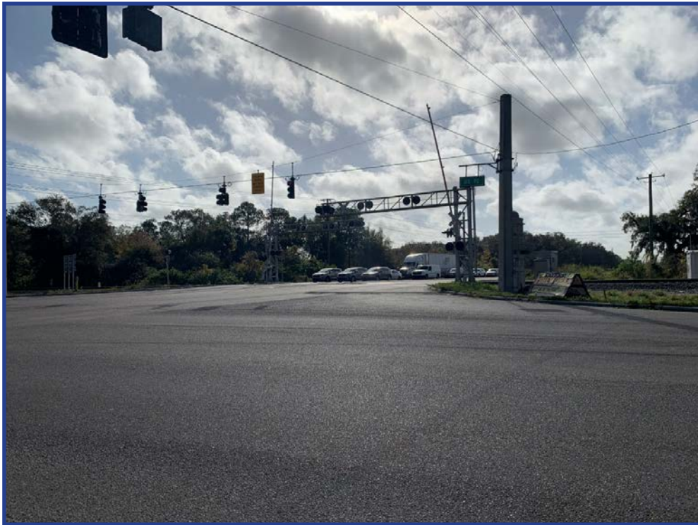
Figure 157: Looking Northwest to US 92
