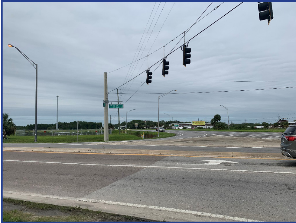
Figure 20: Looking North towards US 27 from Southwest Quadrant of Intersection
