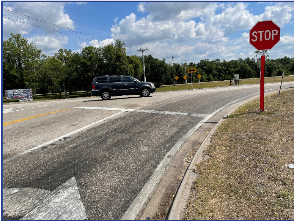
Figure 115: Entering SR 70 from SR 72
