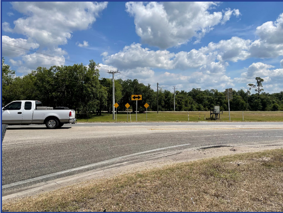
Figure 113: US 27 Looking at Northeast side of the Intersection
