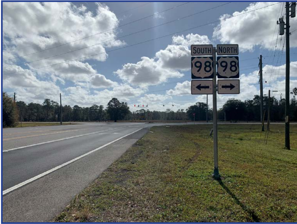
Figure 41: SR 471 Looking South to US 98
