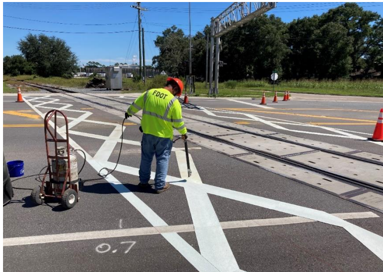
Figure 4-7 | FDOT Staff coating Dynamic Envelope
