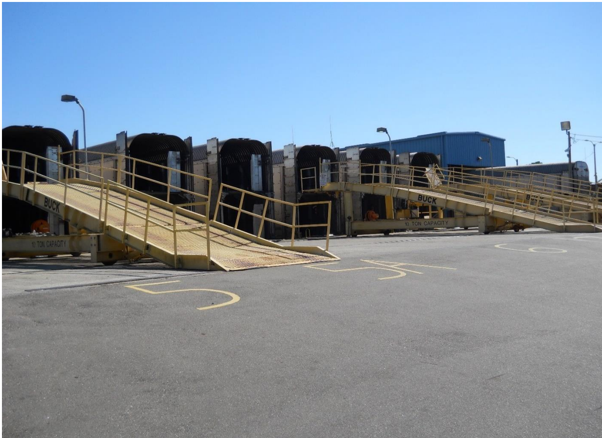
Figure C-3 | Auto Carrying Railcars of Amtrak's Auto Train
