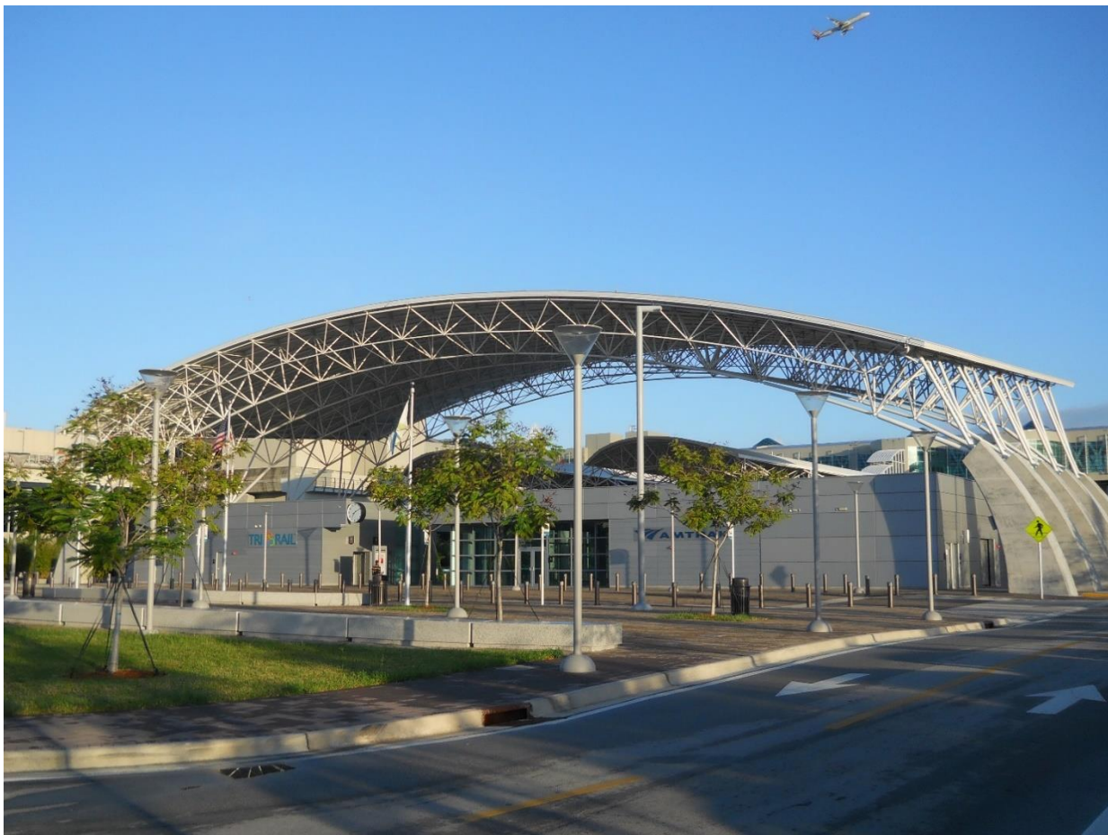
Figure C-5 | Miami Intermodal Center near Miami Airport
