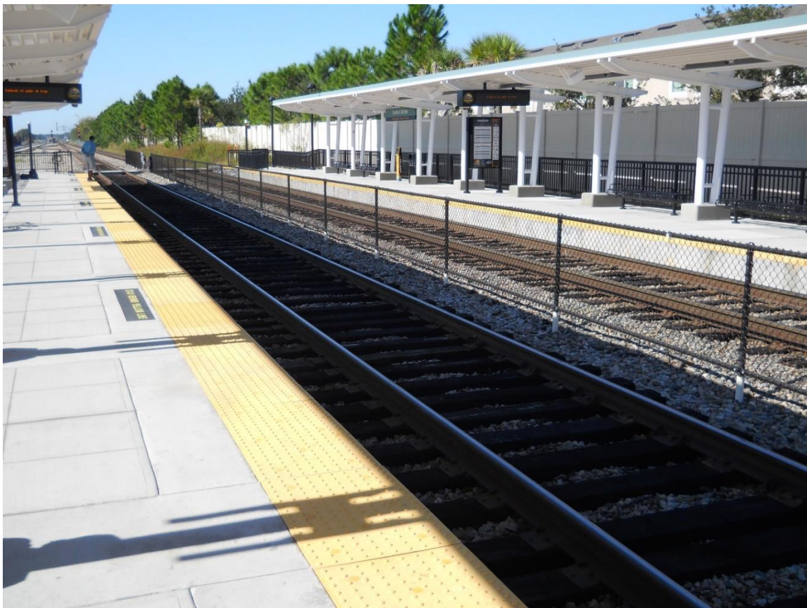
Figure C-10 | Sun Rail's Sanford Station's Double Platform
