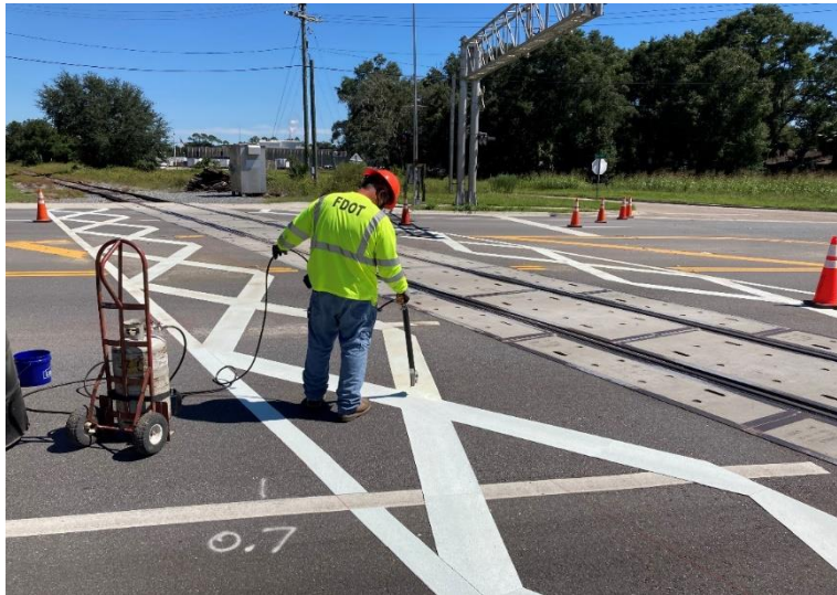
Figure 4-7 | FDOT Staff coating Dynamic Envelope
