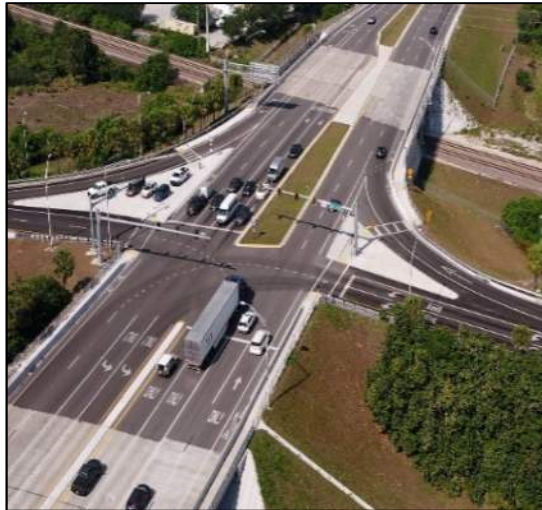
Looking west along Woolbright Road at the I-95 on/off ramps west of the interchange
