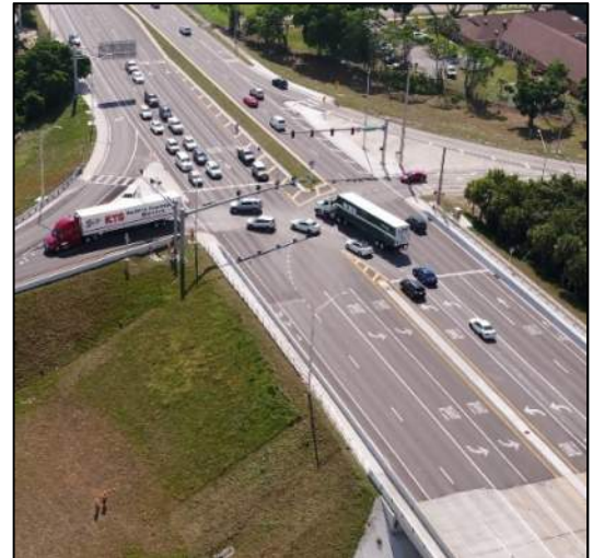
Looking east along Woolbright Road at the I-95 on/off ramps east of the interchange
