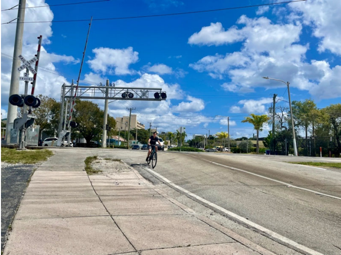
SW 17 th Street with bicyclist west of the train tracks
