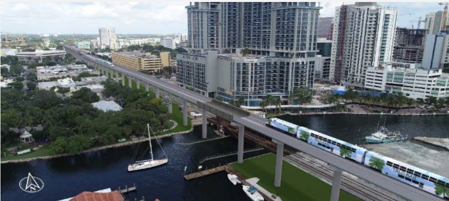
80-foot high-level fixed bridge
