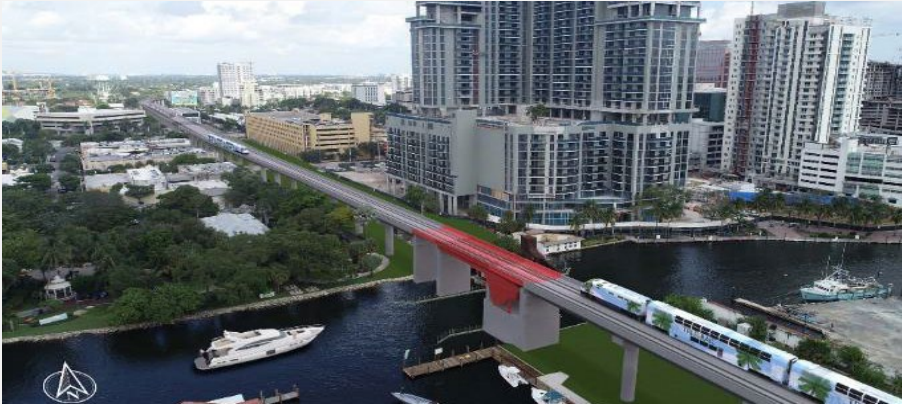
56-foot mid-level bascule
