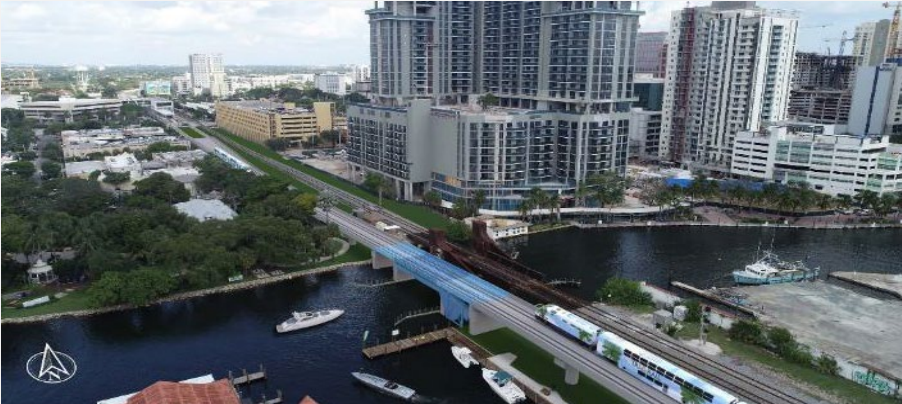
21-foot low-level bascule
