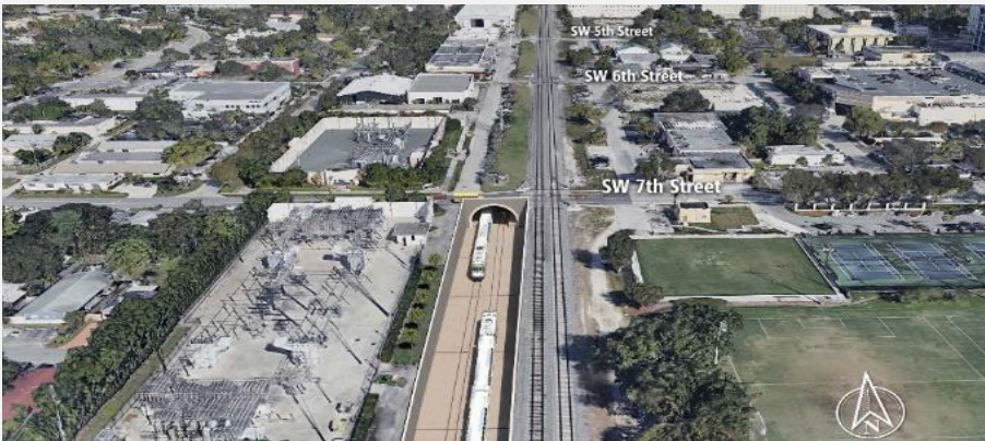
Tunnel beneath New River
