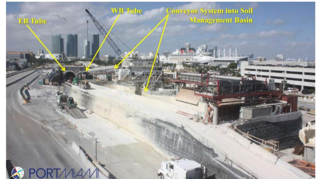
Tunnel Soil Management at Portals
