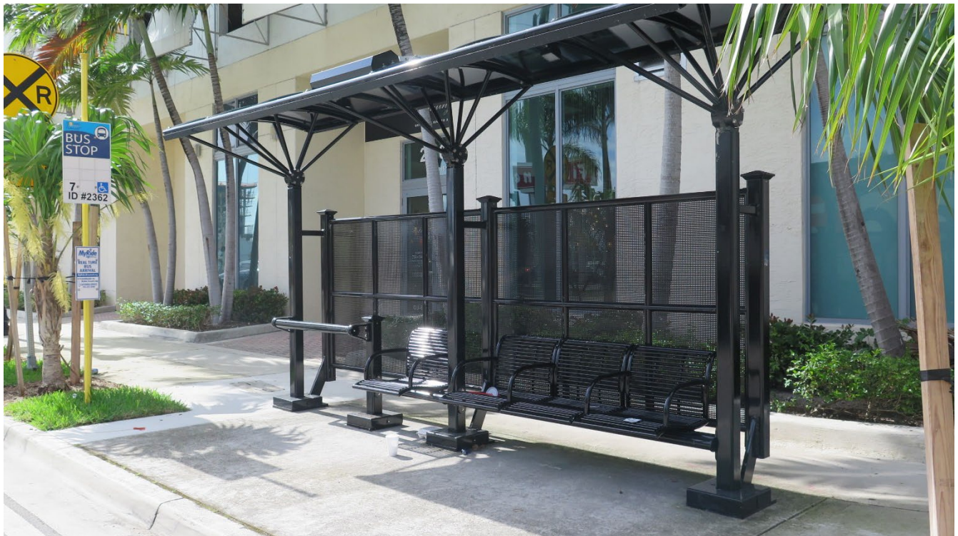
Figure 2-4: Hollywood Boulevard Complete Streets Bus Stop
