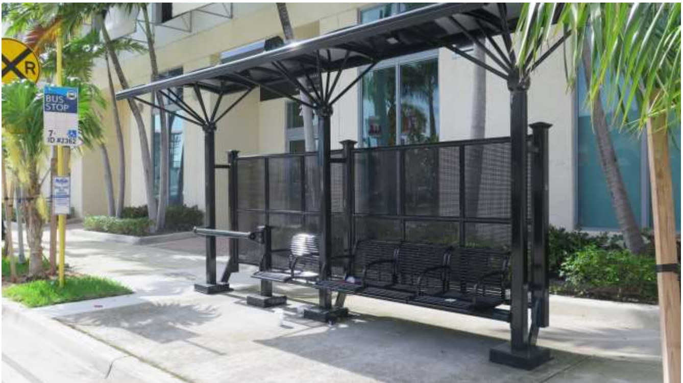
Figure 2-4: Hollywood Boulevard Complete Streets Bus Stop
