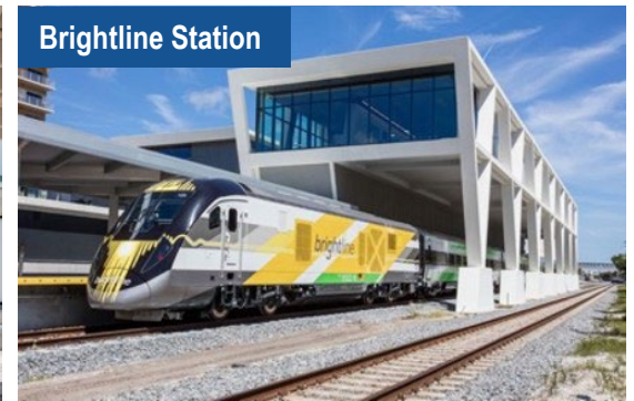
Existing Intercity Passenger Rail Station
