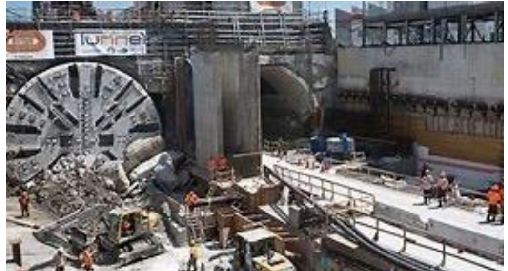
PORT MIAMI TUNNEL BORING MACHINE
