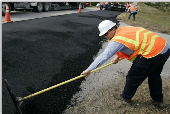
Lake Josephine Road, Highlands County District 1
