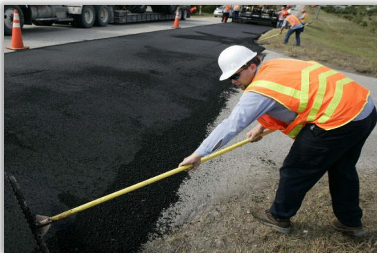
Lake Josephine Road, Highlands County District 1
