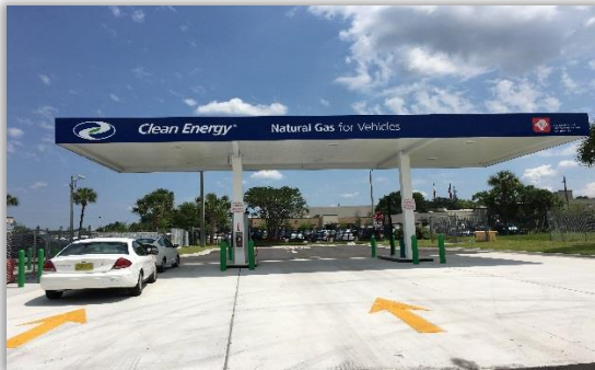
Clean Energy Facilities, Jacksonville Transit Authority TRIP Project, District 2
