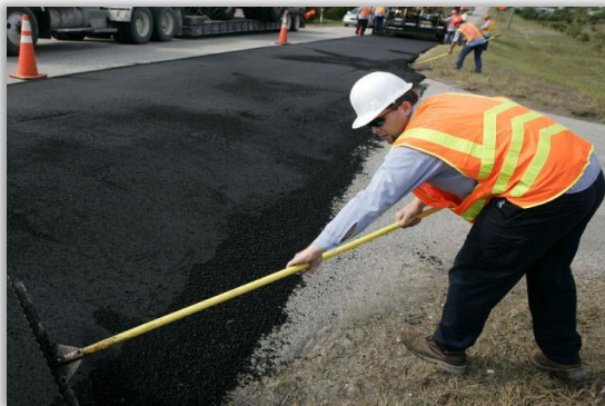
Lake Josephine Road, Highlands County District 1
