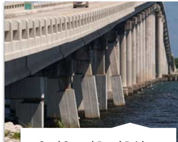
Card Sound Road Bridge, Monroe County SCOP Project
