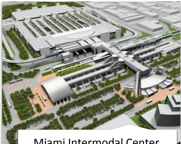
Miami Intermodal Center, Miami Dade County TRIP Project
