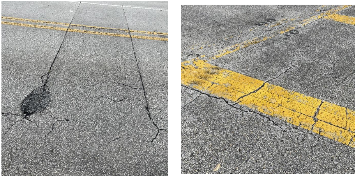
Figure 2-4 Existing Pavement Conditions
