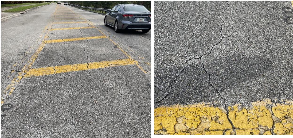
Figure 2-10 Existing Signs and Pavement Markings
