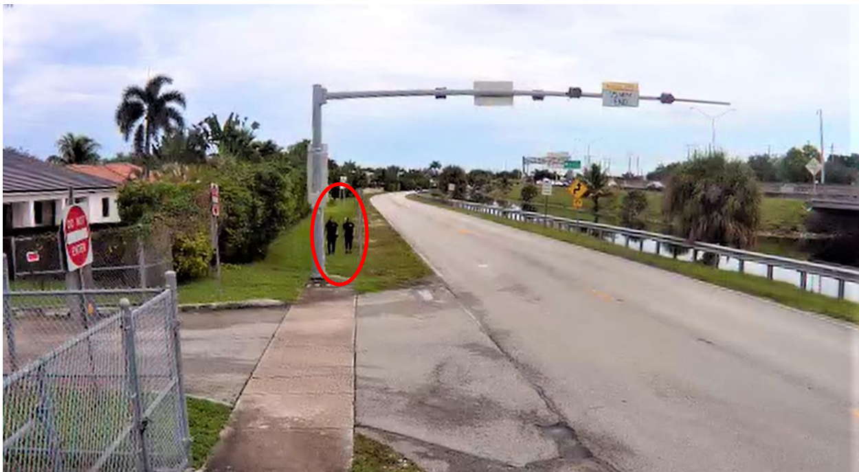
Pedestrians observed walking along the southbound shoulder with no existing sidewalk. The pedestrians were observed coming from the residential community on the northeast side and going to the Royal Oaks Shopping Plaza.
