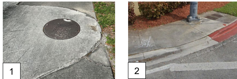
Figure 2-5 Sidewalk Deficiencies
