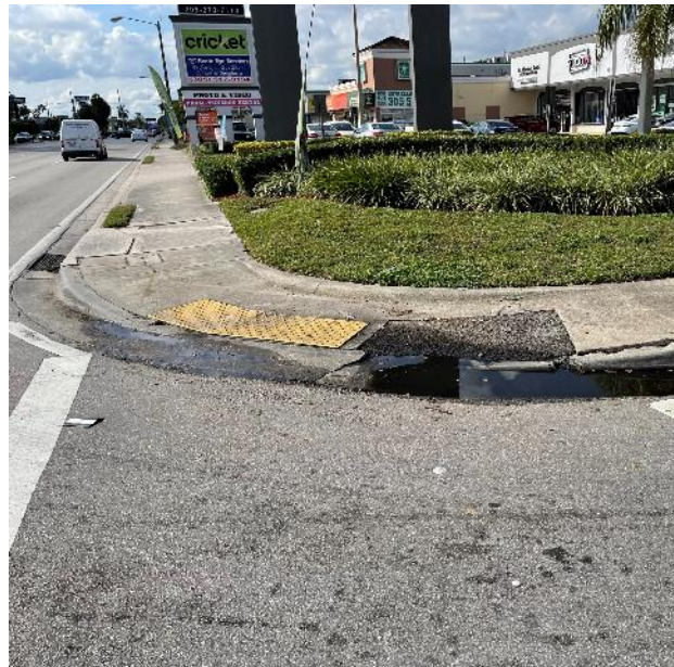
Photo 15: Looking west at the northwest corner of West 12 Lane.
