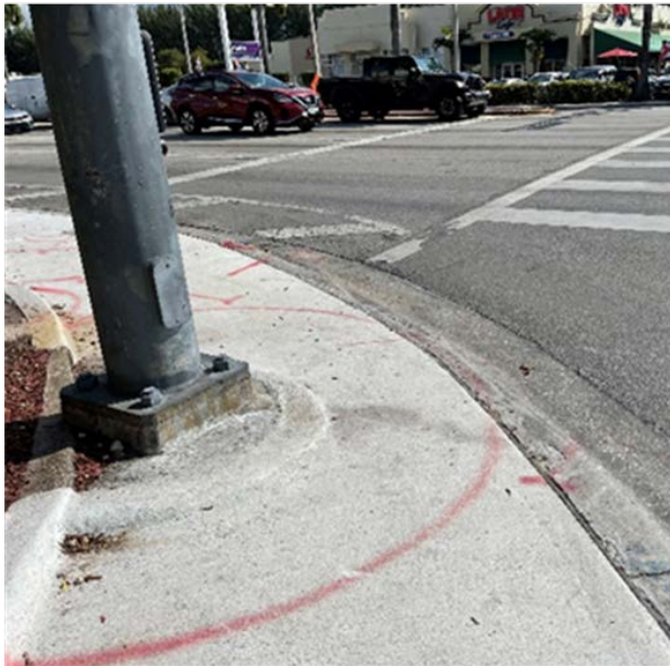
Photo 28: Looking at the northeast corner of West 12 Avenue.
