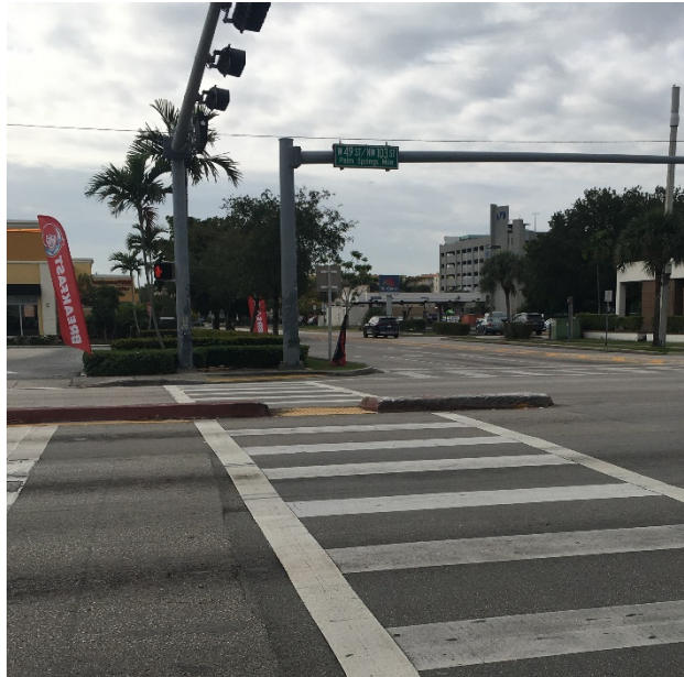
Photo 49: Traffic separator on the east leg crosswalk of West 17 Court.
