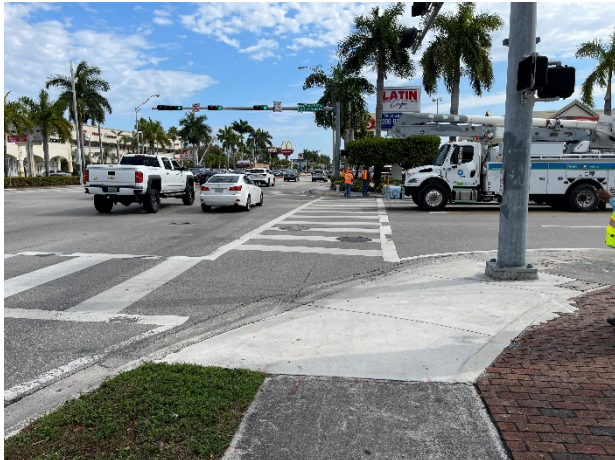
Photo 20: Looking east at the southwest corner of West 12 Avenue.
