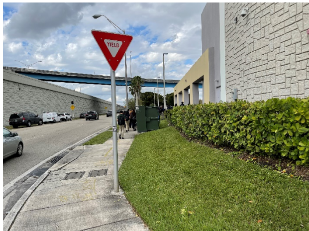
Photo 69: Looking north at the northeast corner of SR 826 East.
