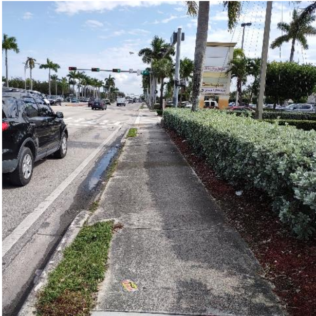
Photo 16: Looking at driveway west of the southwest corner of West 6 Avenue.
