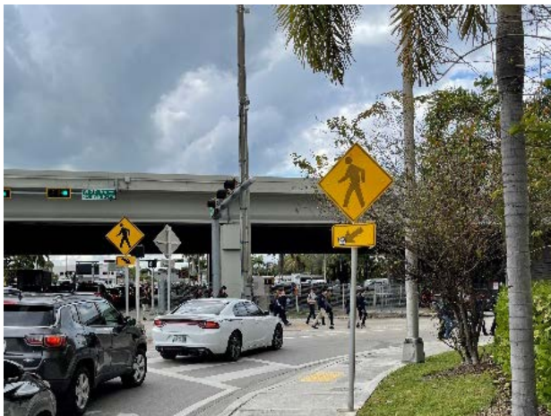
Photo 68: Looking west at the northeast corner of SR 826 East.
