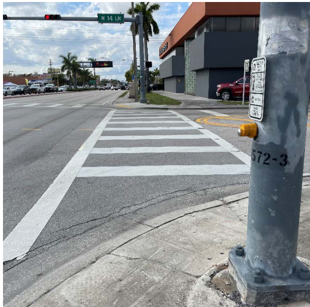
Photo 23: Looking west at the northeast corner of West 14 Lane.
