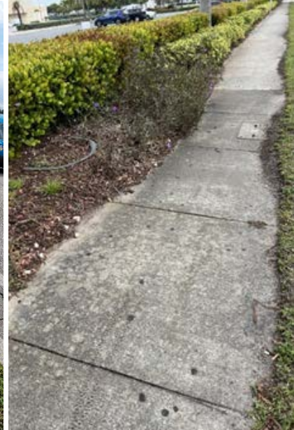
Photo 5: North side sidewalk east of West 17 Court
