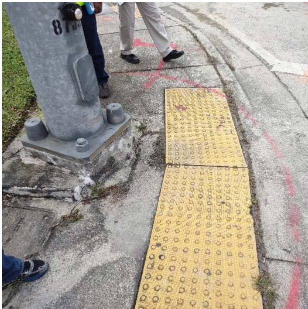
Photo 30: Looking at the northeast corner of West 8 Avenue.
