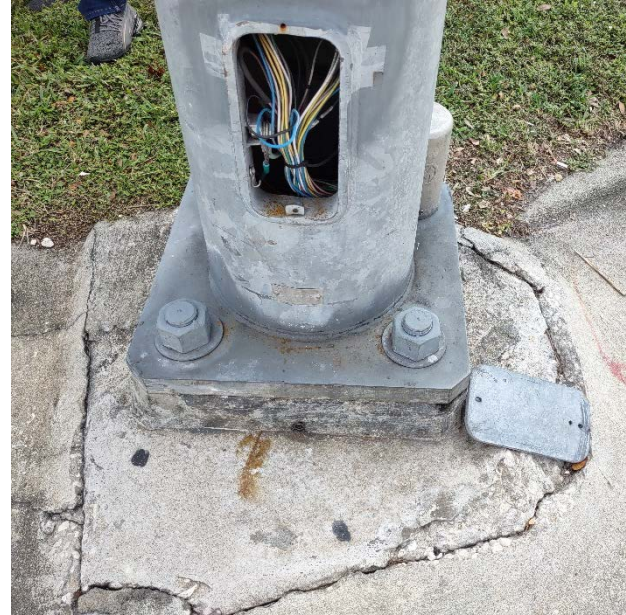
Photo 77: The base of the mast arm on the southeast corner.
