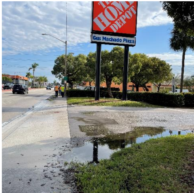
Photo 13: Looking east at the southwest corner of the driveway east of West 16 Avenue.
