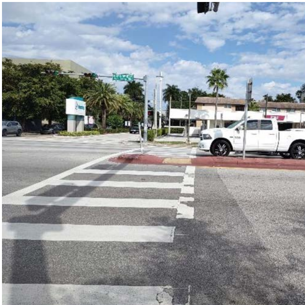
Photo 50: Traffic separator on the east leg crosswalk of West 14 Lane.
