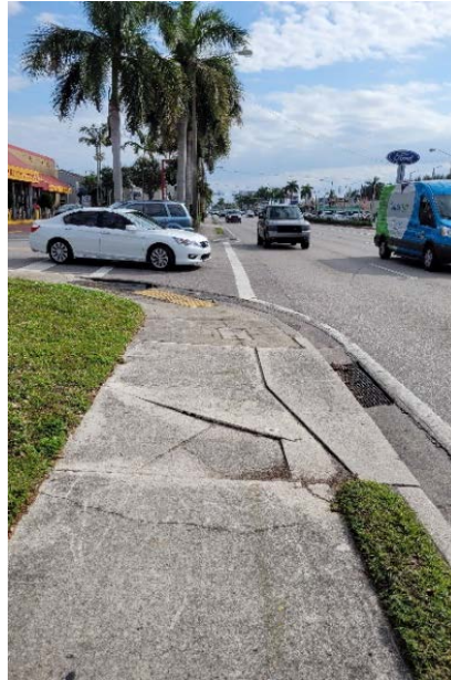
Photo 4: Looking at the northwest corner of West 12 Lane.
