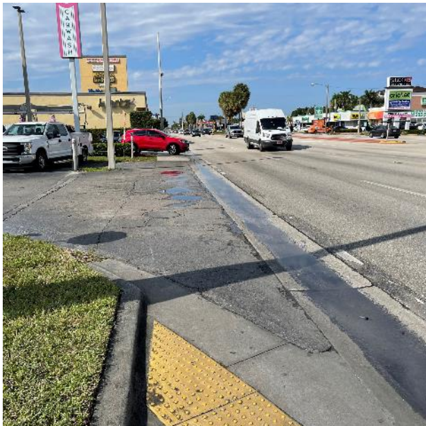
Photo 14: Looking west at the southeast corner of West 12 Lane.
