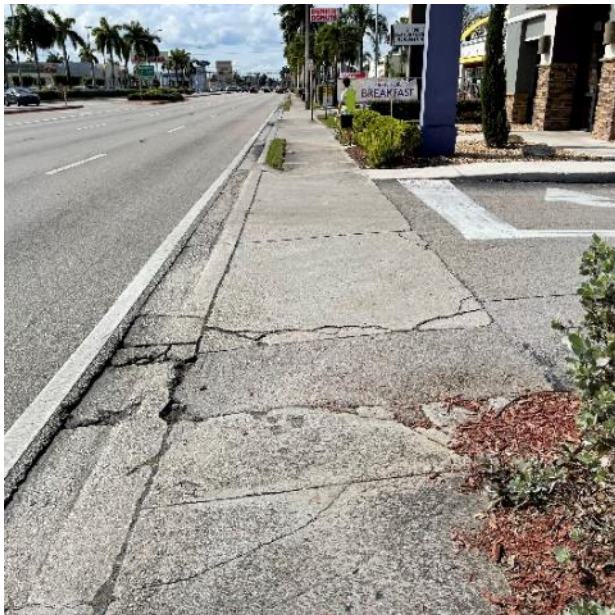
Photo 18: Looking west at the Taco Bell driveway west of the northwest corner of West 10 Avenue.
