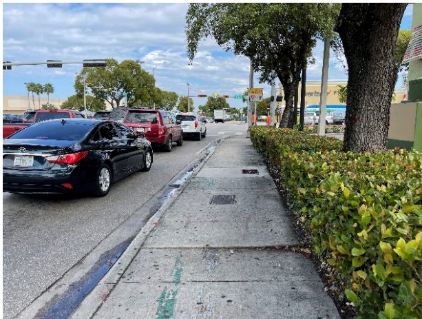
Photo 6: East side sidewalk approaching the southeast corner of West 16 Avenue.
