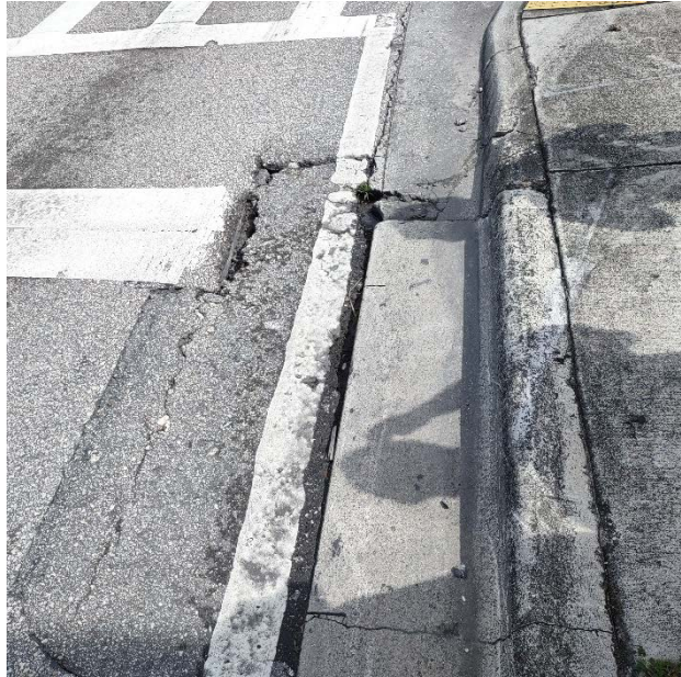
Photo 79: Eastbound outside lane approaching the intersection.
