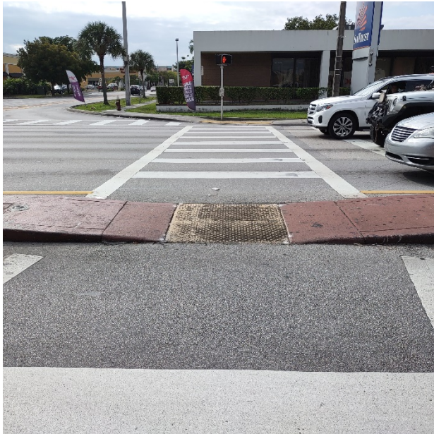
Photo 48: Traffic separator on the west leg crosswalk of West 17 Court.
