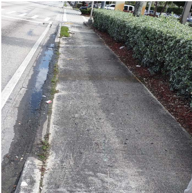
Photo 80: Driveway on the south side west of the intersection.
