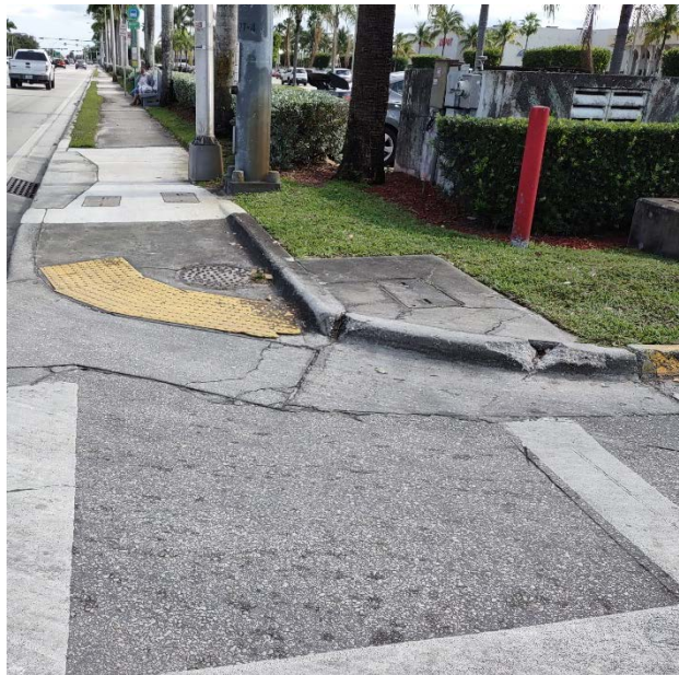
Photo 81: Pedestrian ramp at the southeast corner.
