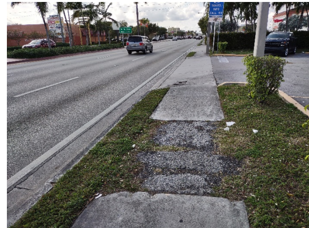
Photo 7: North side sidewalk west of West 14 Lane.
