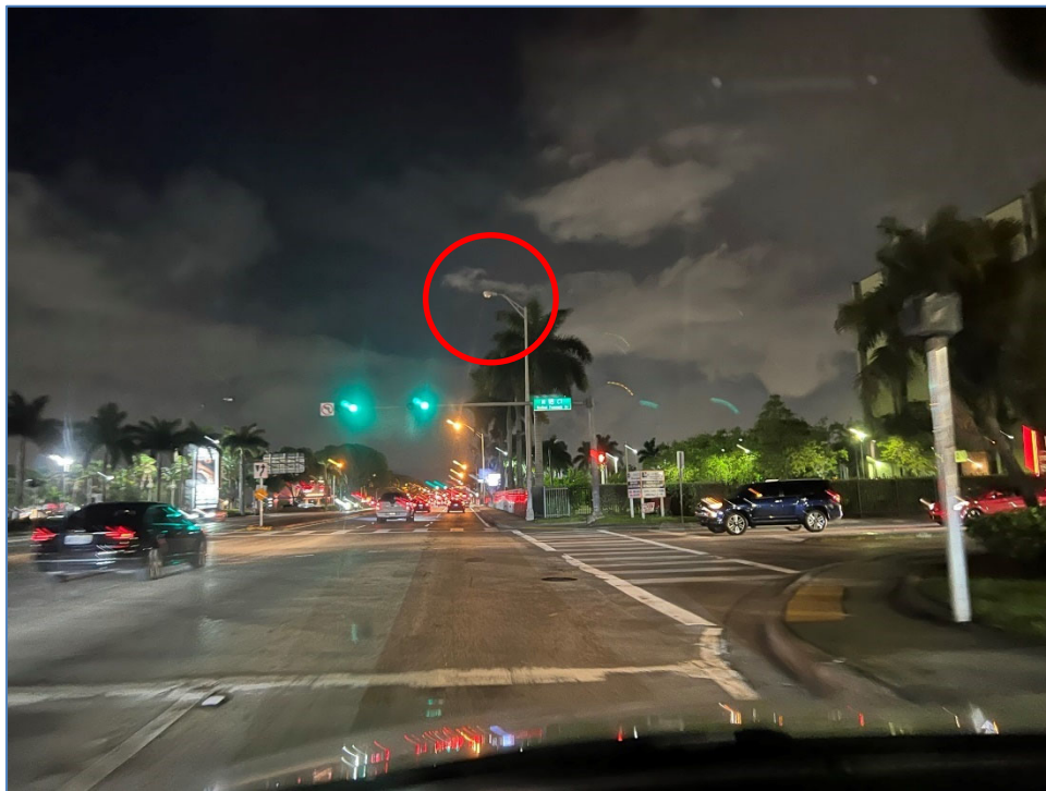
Photo 3 – Non-functioning luminaire east of W 18 th Ct (south side of SR 932/NW 103 rd Street)
