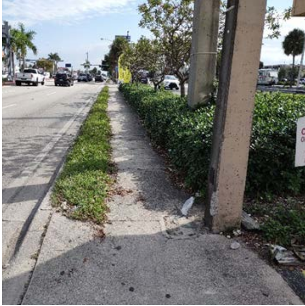
Photo 60: Looking east on the south side sidewalk west of West 14 Lane.
