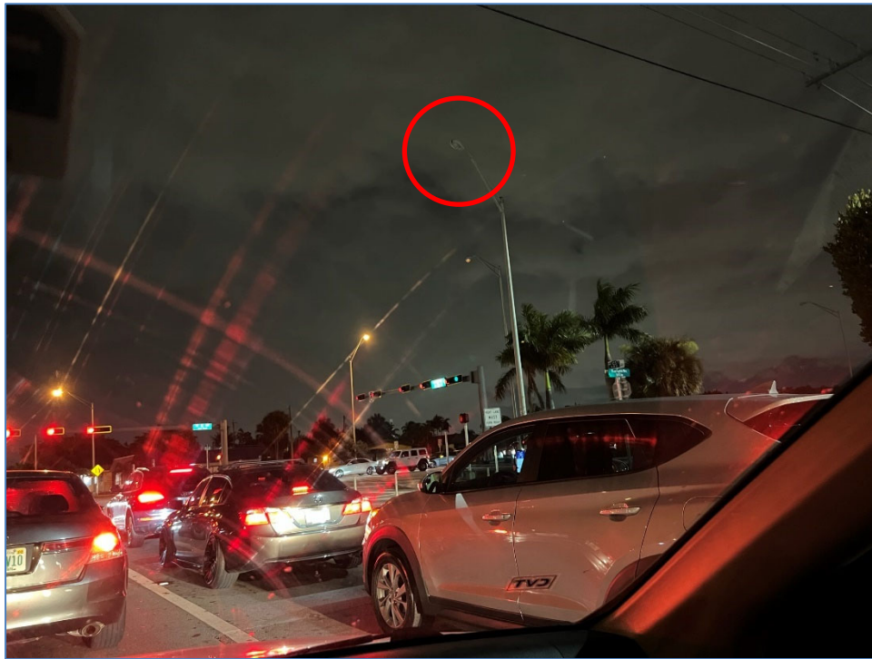
Photo 8 – Non-functioning luminaire east of W 4 th Ave (south side of SR 932/NW 103 rd Street)
