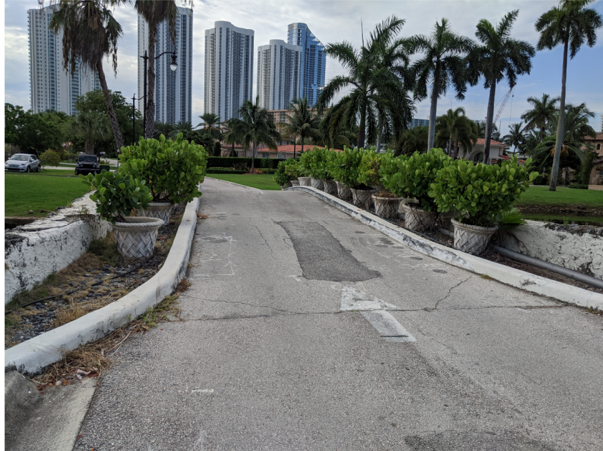
Figure 3: Overall Bridge Deck View – Looking East
