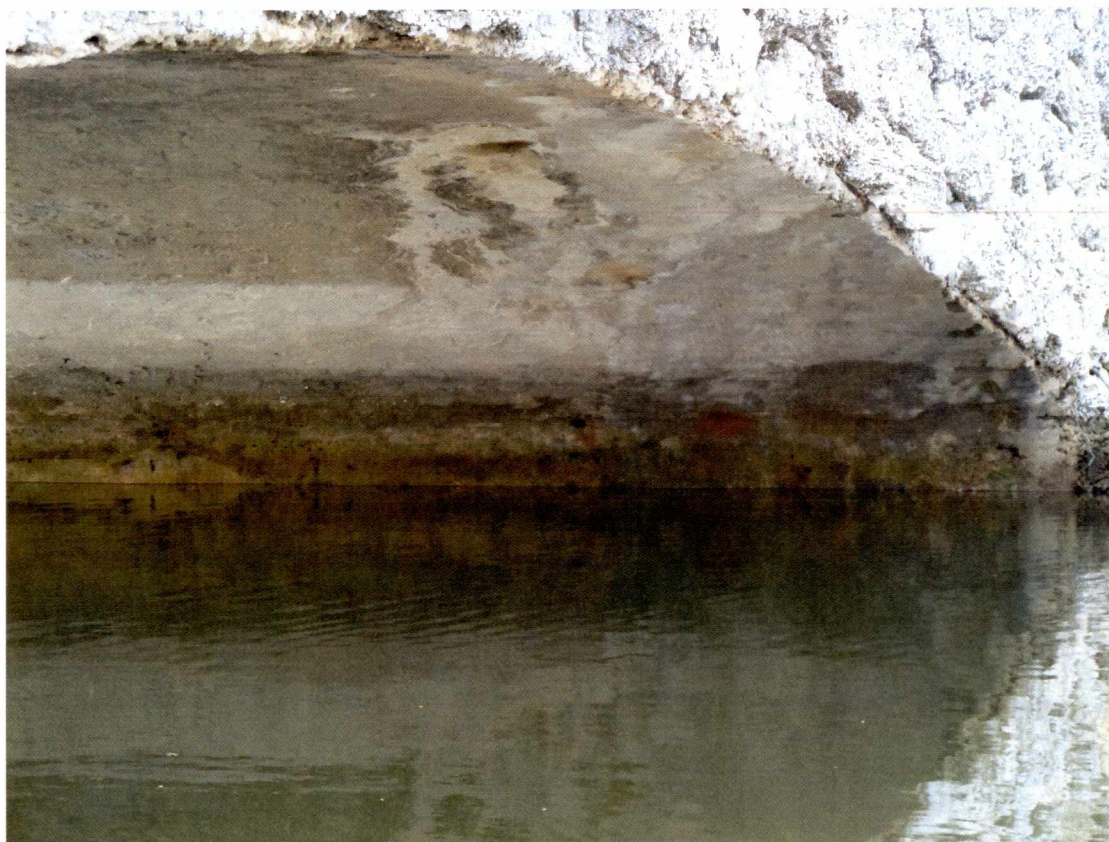
UNDER BRIDGE VIEW
