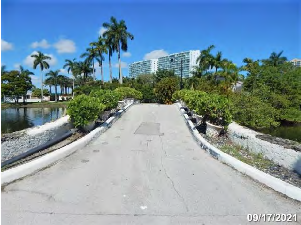
East Approach Looking West - 09/17/2021
