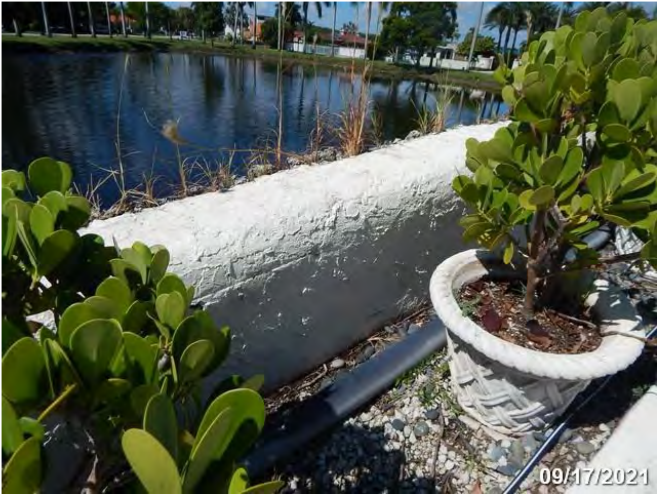
Typical Bridge Rail - 09/17/2021
