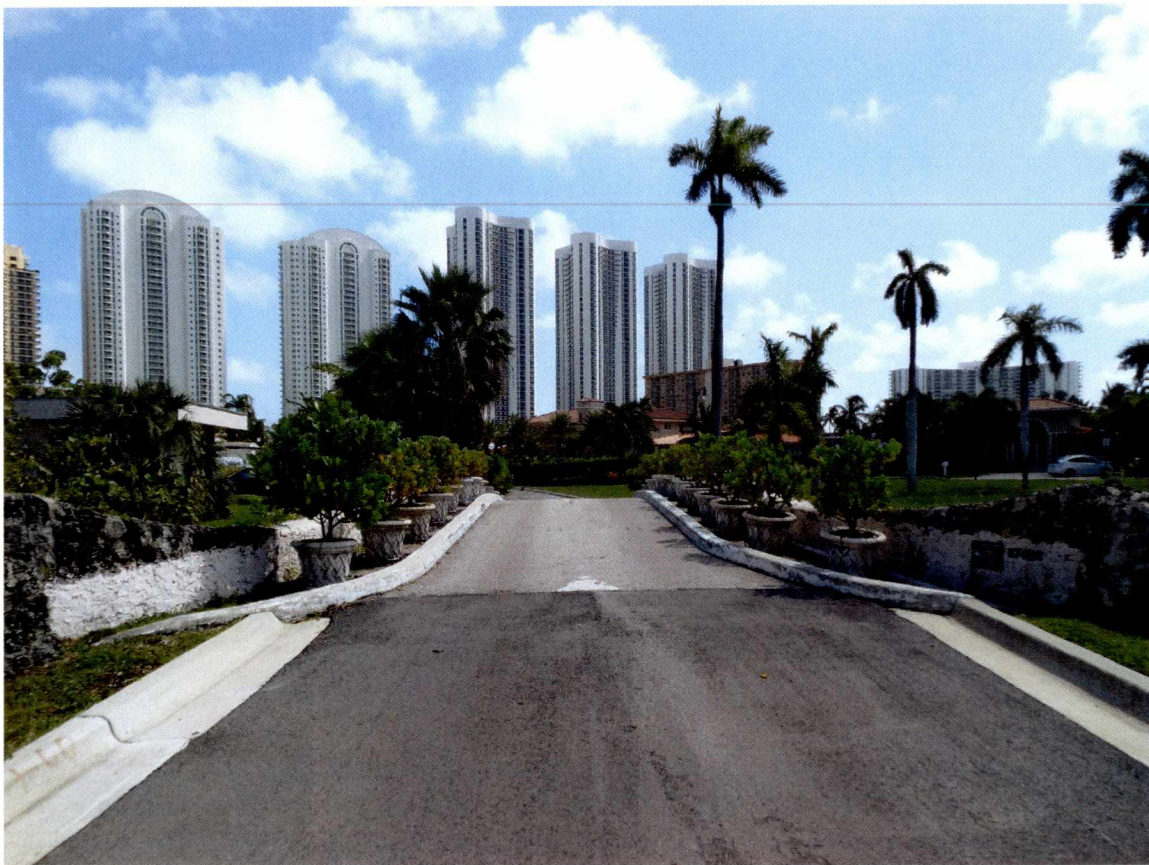
EAST APPROACH OF BRIDGE
