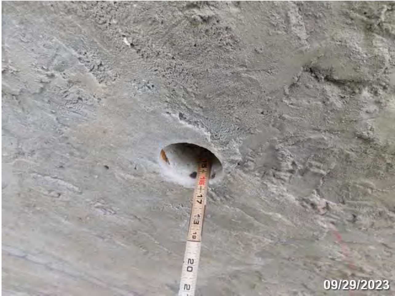
PHOTO 11: ELEMENT/ENV: 144/4 Re Conc Arch
