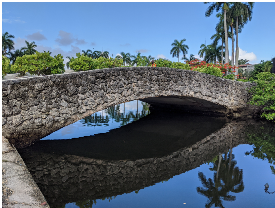
Figure 4: Overall Bridge Elevation View – Looking Southwest
