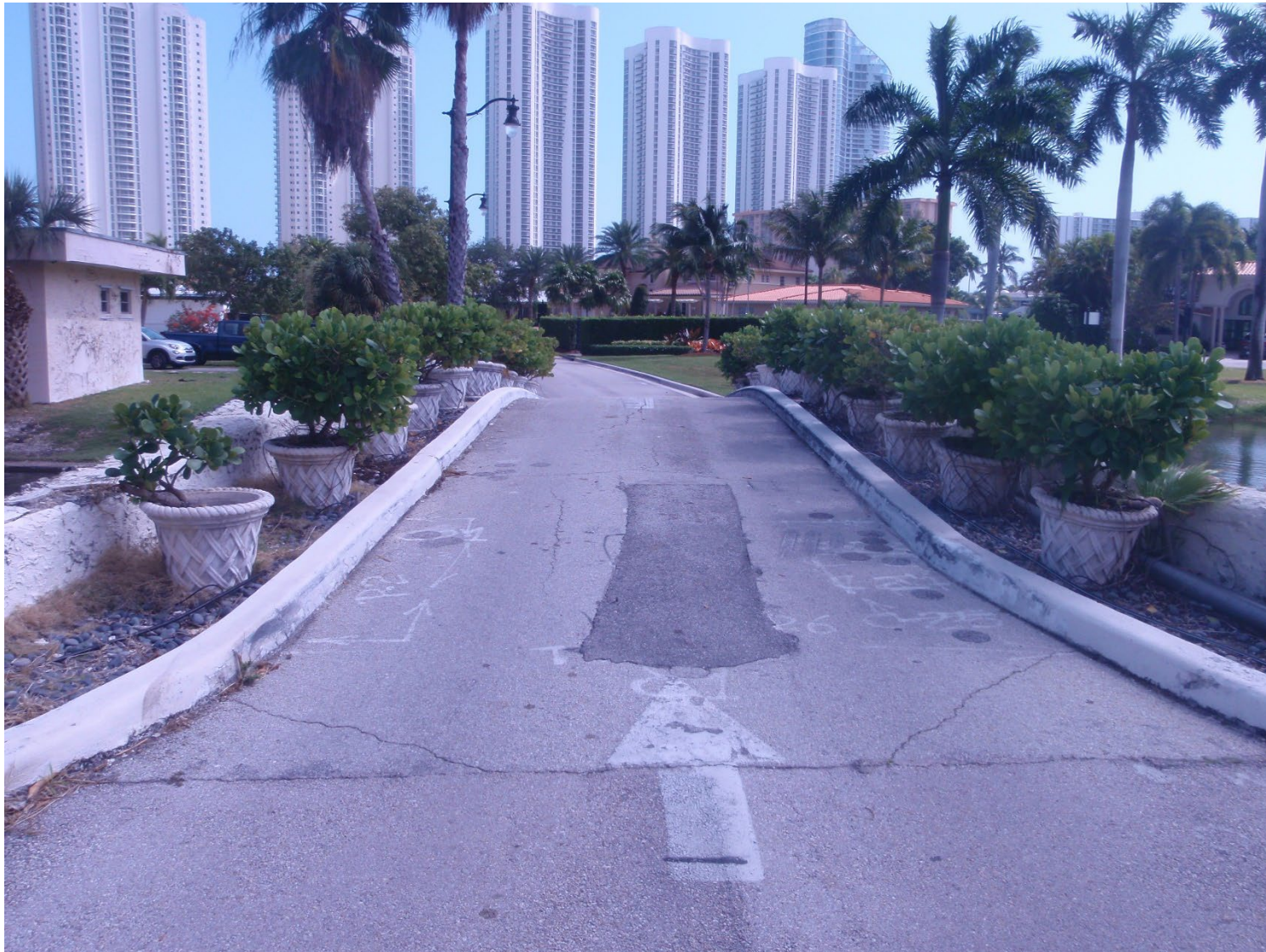
Figure 2-8. Existing Planter Easement Along Bridge
