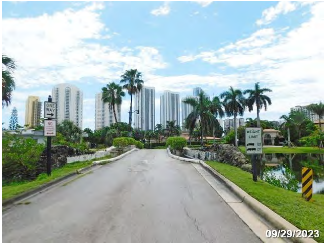
PHOTO 8: ELEMENT/ENV: 144/4 Re Conc Arch
