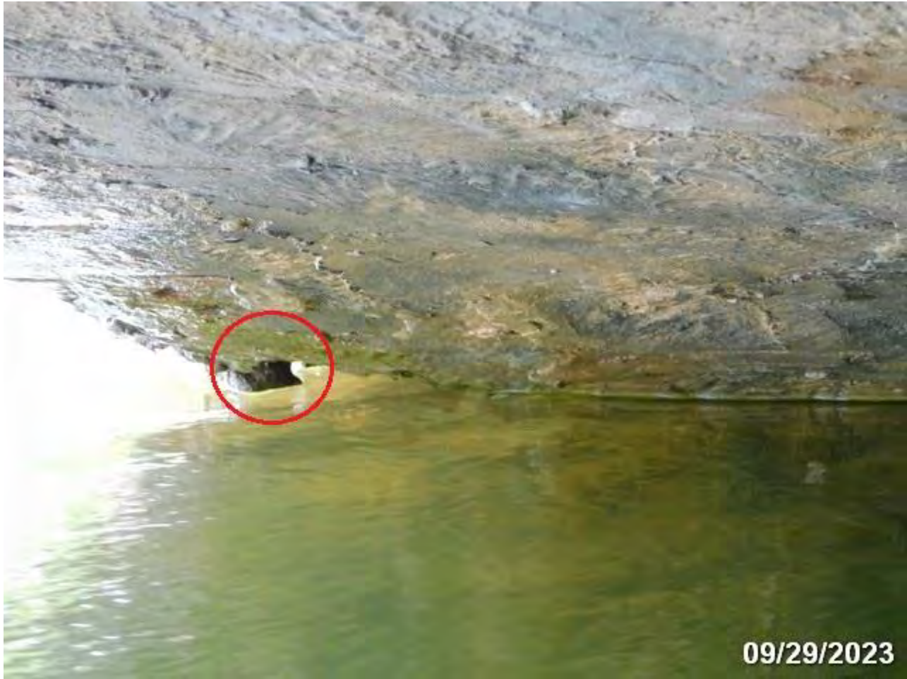
PHOTO 12: ELEMENT/ENV: 144/4 Re Conc Arch
