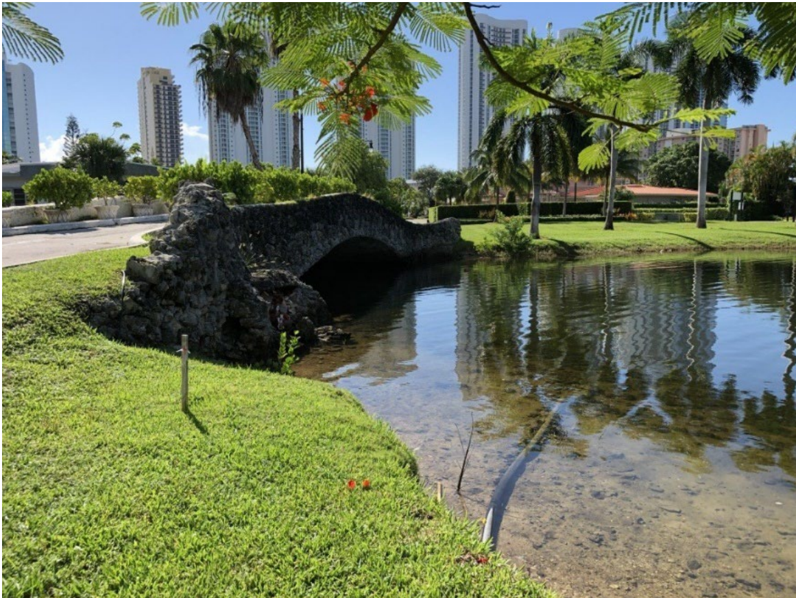
Figure 2-9. Atlantic Isle Lagoon Bridge – Southeastern View
