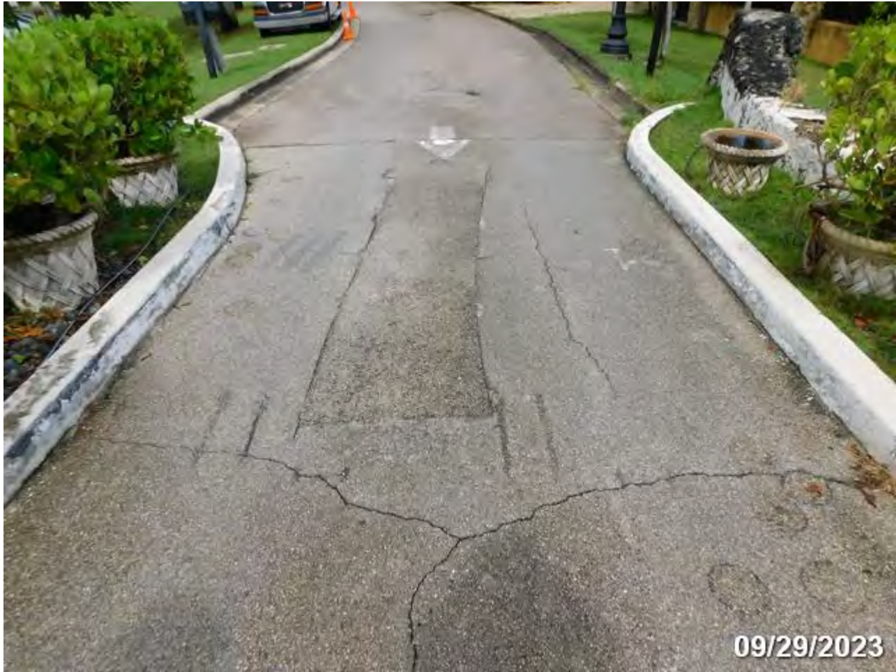
PHOTO 5: ELEMENT/ENV: 144/4 Re Conc Arch
