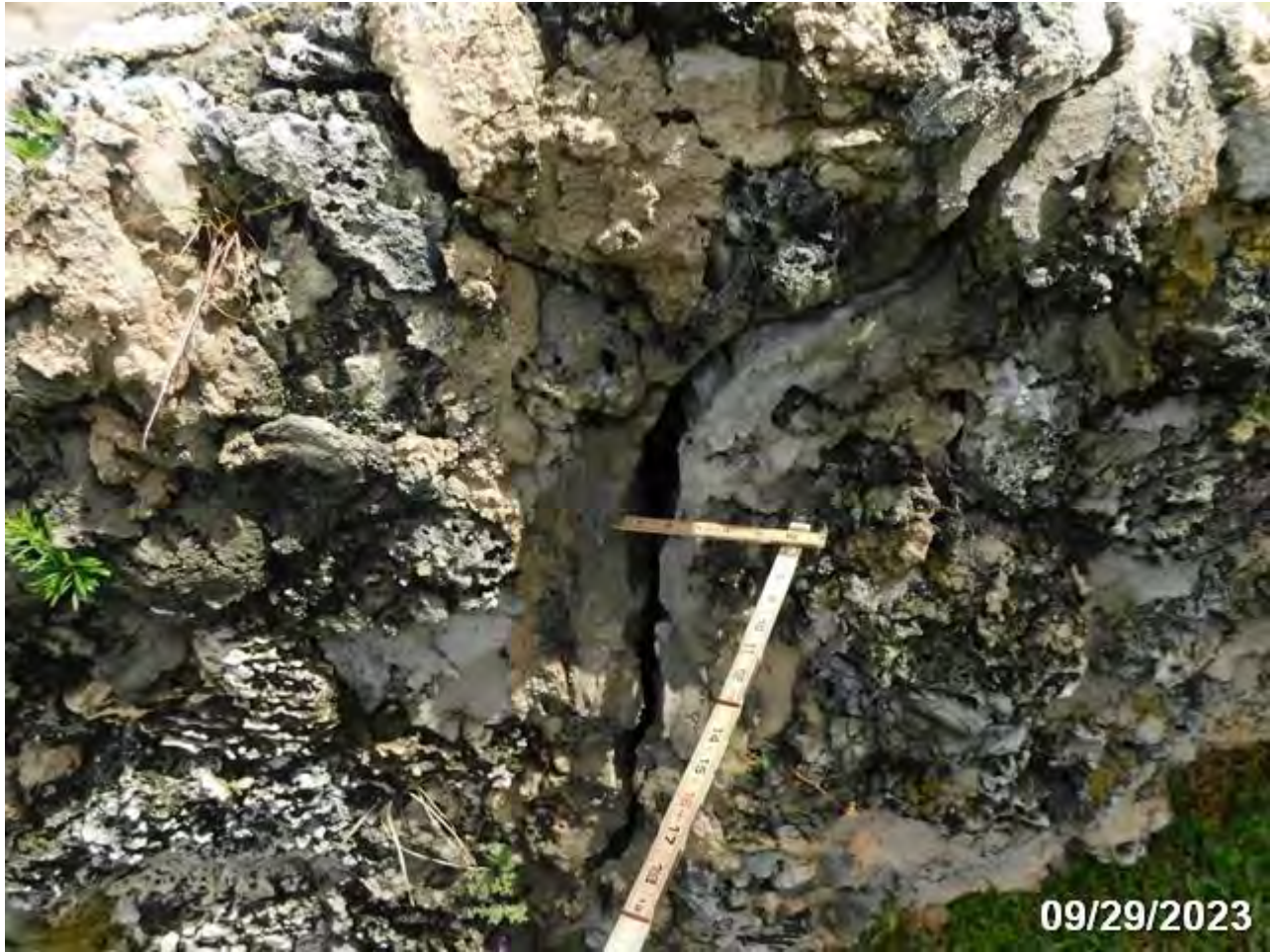
PHOTO 2: ELEMENT/ENV: 8477/4 Other Wingwalls/Retaining Wall
