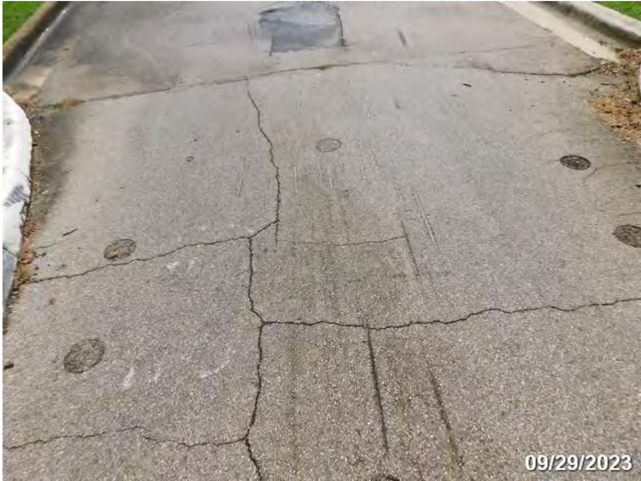
PHOTO 6: ELEMENT/ENV: 144/4 Re Conc Arch
