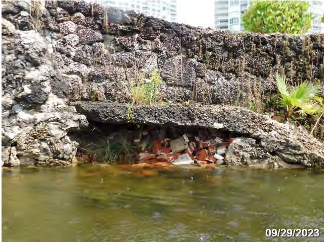
PHOTO 3: ELEMENT/ENV: 8477/4 Other Wingwalls/Retaining Wall
