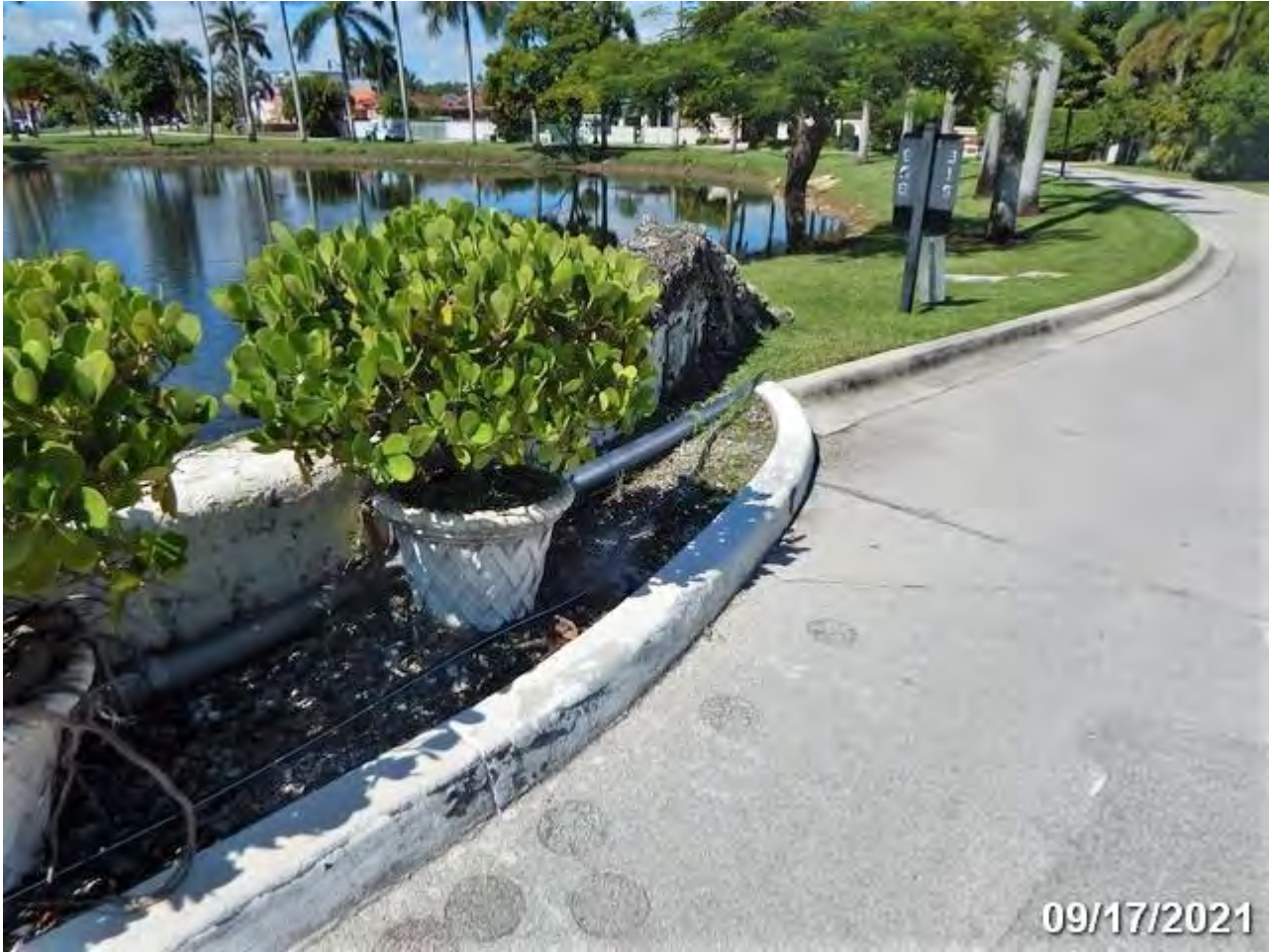
Southwest Oncoming Transition - 09/17/2021
