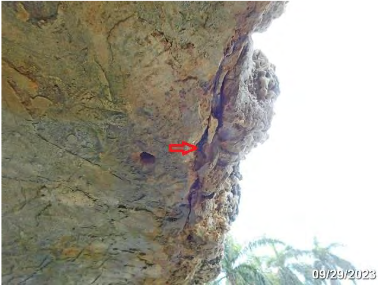
PHOTO 10: ELEMENT/ENV: 144/4 Re Conc Arch
