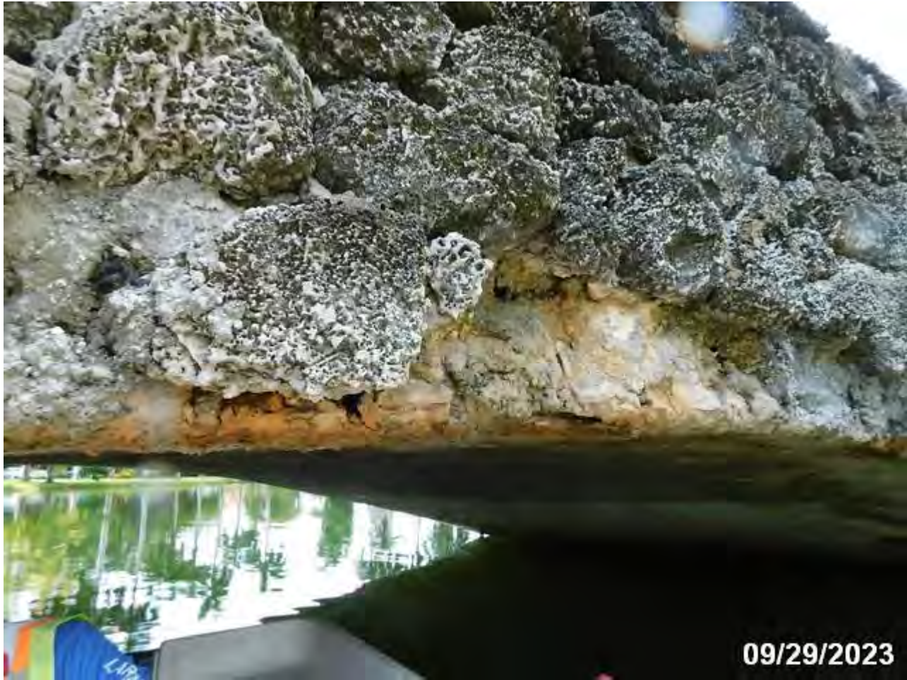
PHOTO 7: ELEMENT/ENV: 144/4 Re Conc Arch
