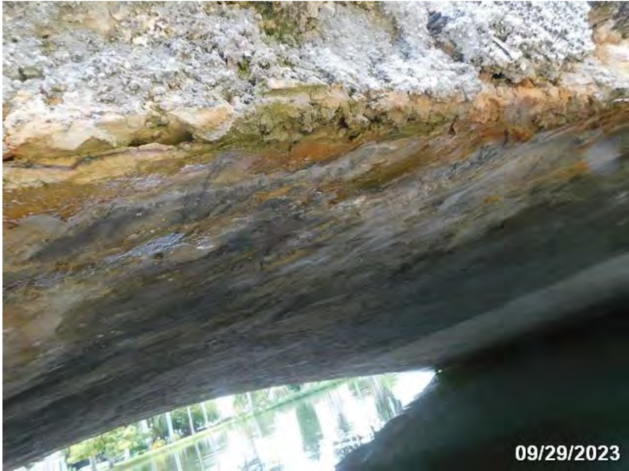
PHOTO 9: ELEMENT/ENV: 144/4 Re Conc Arch
