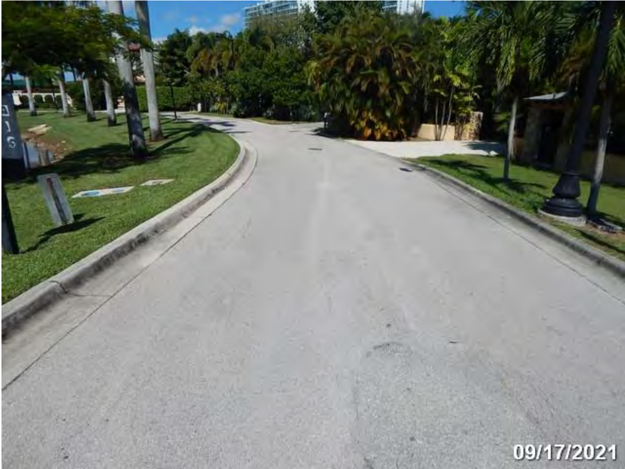
West Approach Looking West - 09/17/2021
