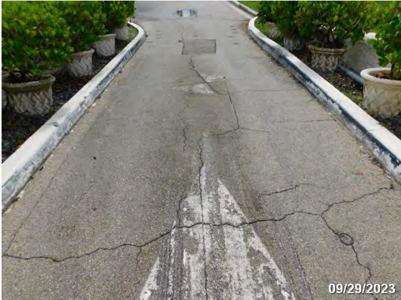
PHOTO 4: ELEMENT/ENV: 144/4 Re Conc Arch
