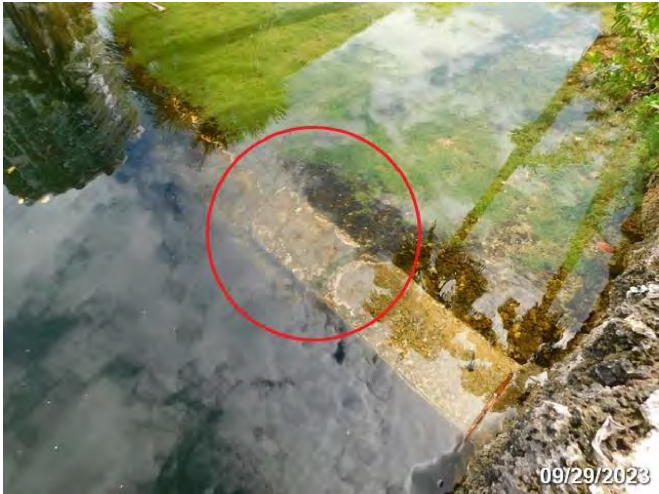
PHOTO 1: ELEMENT/ENV: 8477/4 Other Wingwalls/Retaining Wall
