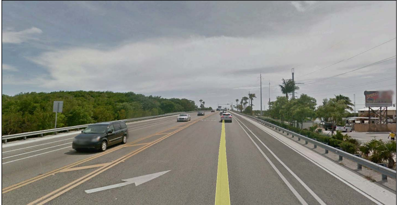
d)- Looking south along southbound SR 5/US 1, approximately 950 ft north from center of bridge (Image date: July 2015).
