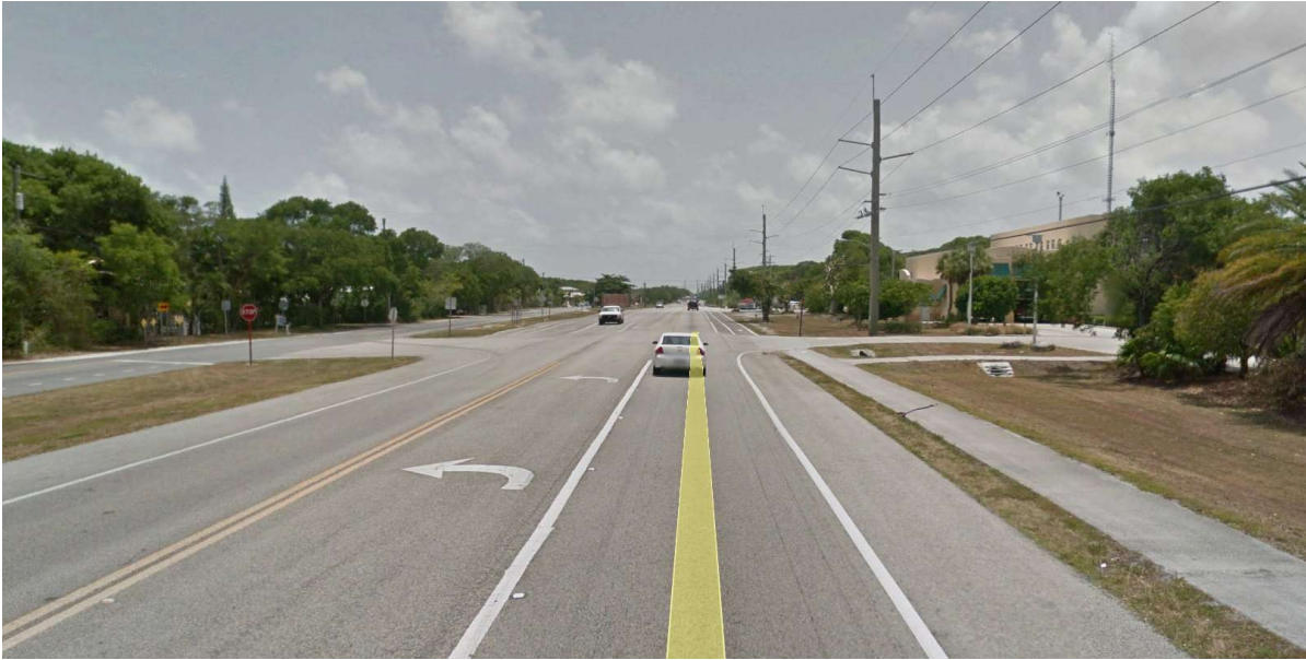
b)- Looking south along southbound SR 5 approximately 150 feet north of fatal crash location (Image date: July 2015).
