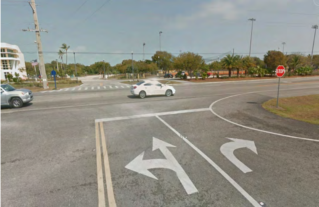
c)- Looking west along westbound approach of the study intersection (Image date: March 2015)
