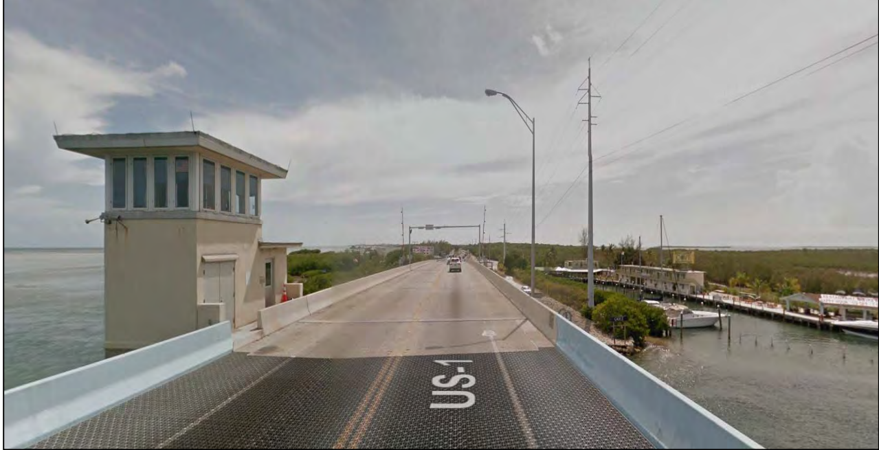
b)- Looking south along southbound SR 5/US 1, approximate subject fatal crash location (Image date: July 2015).
