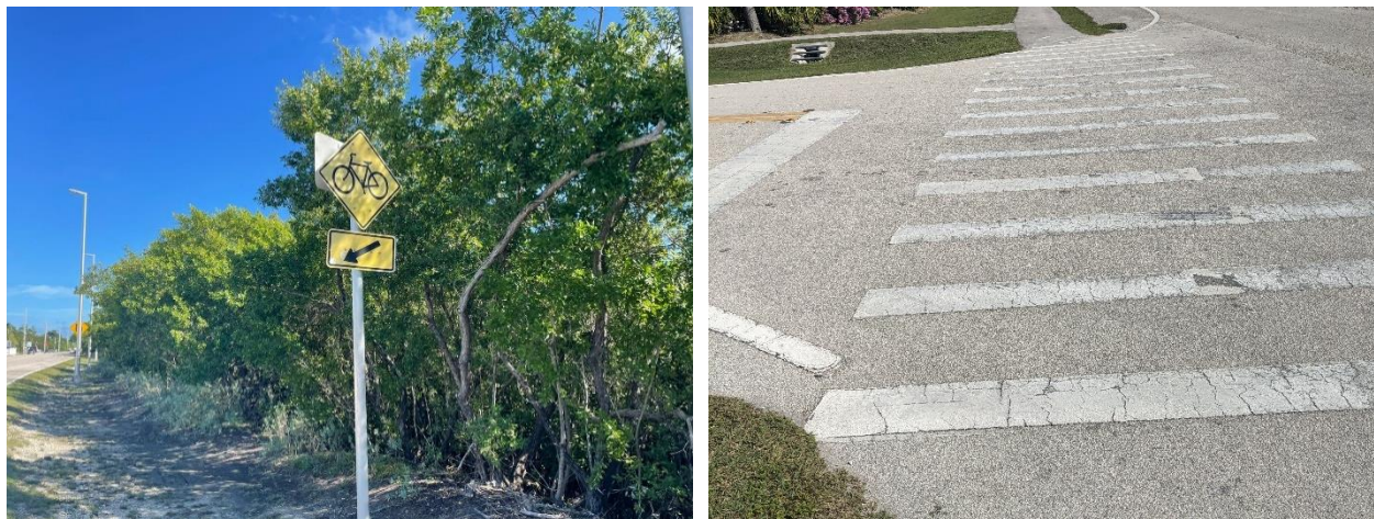
Figure 2-9 Existing Signs and Pavement Markings
