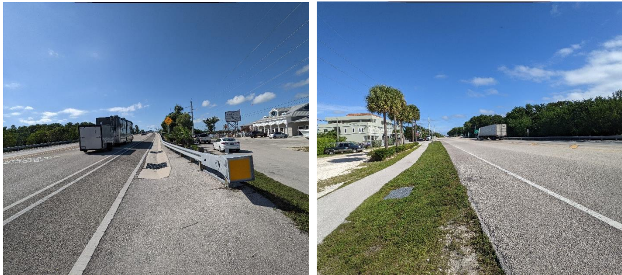
Figure 2-7 Existing Drainage System
