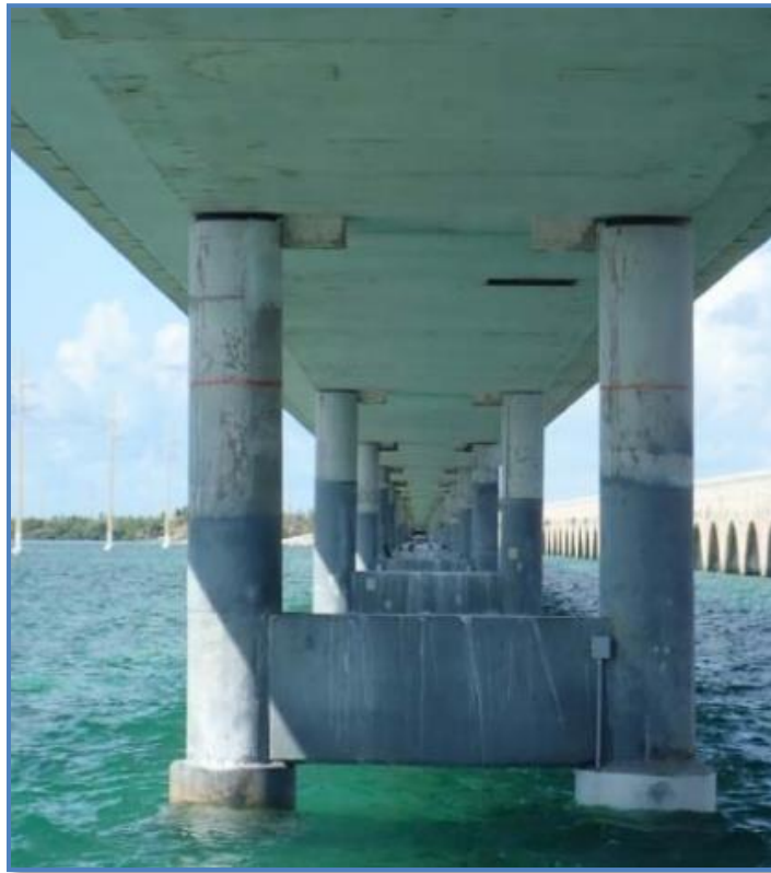
Figure 3-2 View of Bridge Low Span Section
