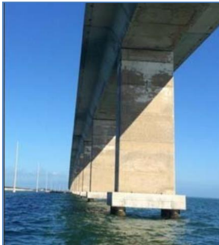
Figure 3-3 View of Bridge High Span Section
