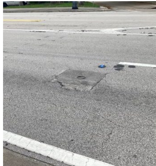
2. UTILITY PATCH ON ASPHALT
