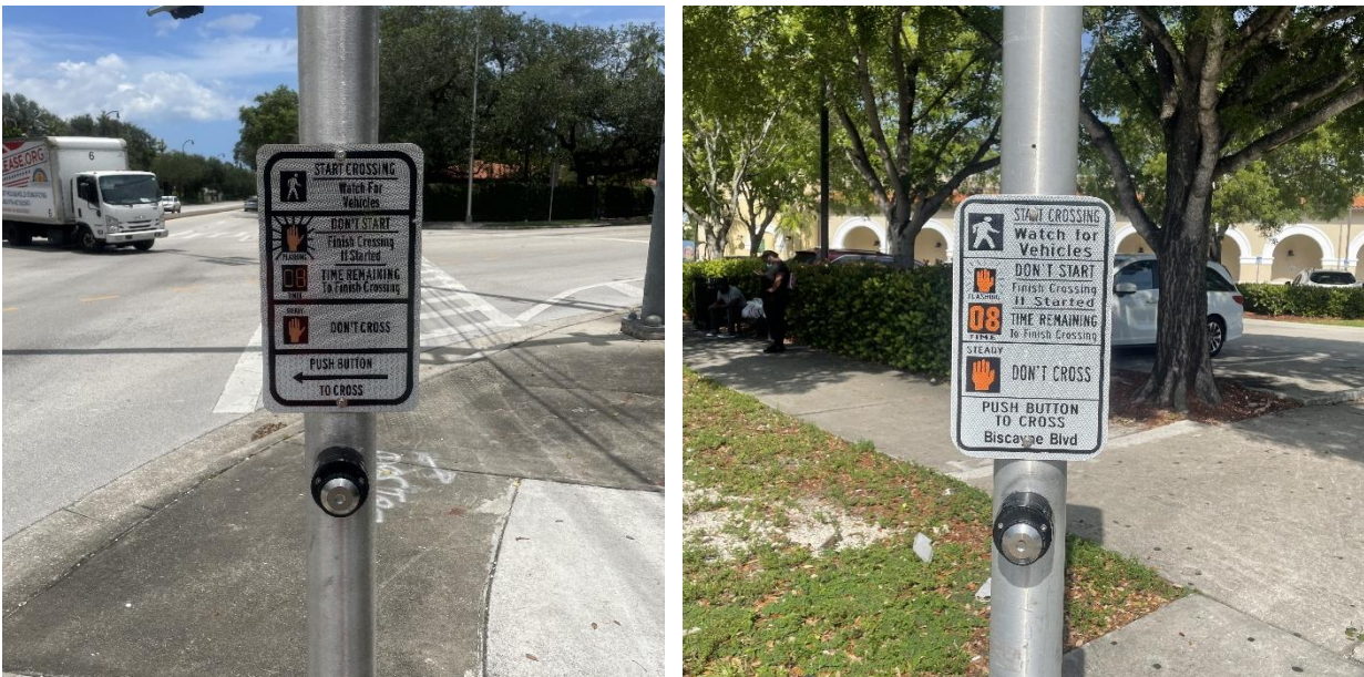
Figure 2-10 Existing Pedestrian Signalization Features
