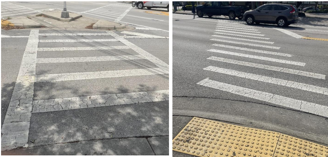
Figure 2-12 Existing Signs and Pavement Markings
