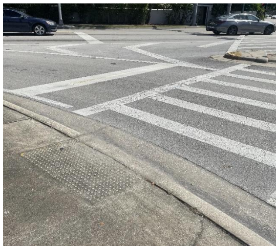
Figure 2-9 Existing Curb Ramps
