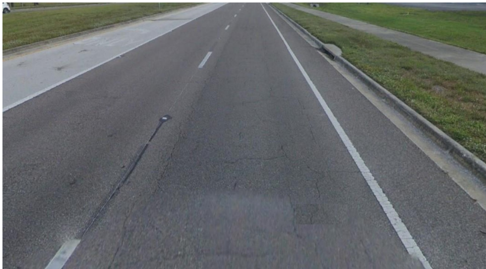
Figure 2: Existing median and outside Type F curb and 4-ft offset from the EOTW to the outside gutter lip on southbound SR 35. The inside lane is a left turn.
