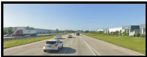
End Project MP 23.836 SLD 12075.000 Southbound, looking south
