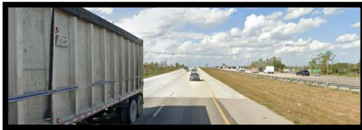
Begin Project MP 22.397 SLD 12075.000 Southbound, looking north
