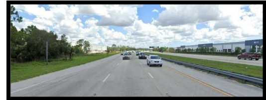
End Project MP 23.836 SLD 12075.000 Northbound, looking south
