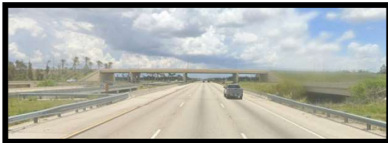
Begin Project MP 13.882 SLD 12075.000 Southbound, looking north
