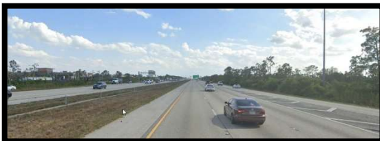
End Project MP 16.100 SLD 12075.000 Southbound, looking south
