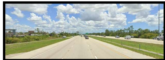
End Project MP 16.100 SLD 12075.000 Northbound, looking south
