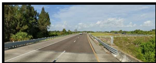
Begin Resurfacing MP 3.884 SLD 13175.000 Southbound, looking north
