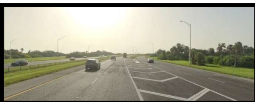
End Project MP 5.233 SLD 13175.000 Southbound, looking south
