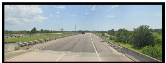
Begin Resurfacing MP 3.884 SLD 13175.000 Northbound, looking north
