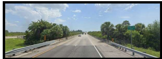
Begin Project MP 3.553 SLD 13175.000 Northbound, looking north
