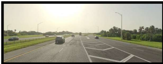
End Project MP 5.233 SLD 13175.000 Southbound, looking south
