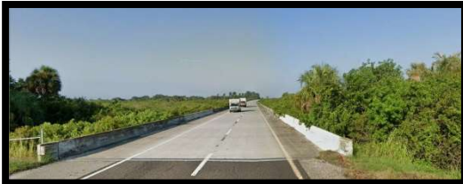
Begin Project MP 3.553 SLD 13175.000 Southbound, looking north
