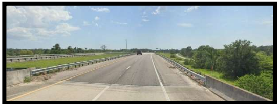
Begin Resurfacing MP 3.884 SLD 13175.000 Northbound, looking north
