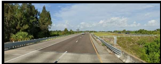
Begin Resurfacing MP 3.884 SLD 13175.000 Southbound, looking north
