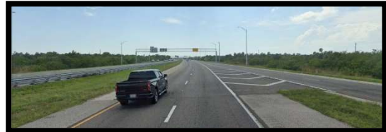
Begin Project MP 9.194 SLD 13130.000 Northbound, looking north
