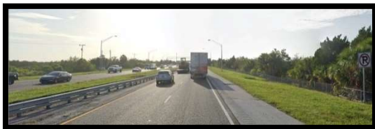
End Project MP 10.005 SLD 13130.000 Southbound, looking south
