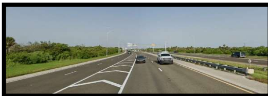
Begin Project MP 9.194 SLD 13130.000 Southbound, looking north
