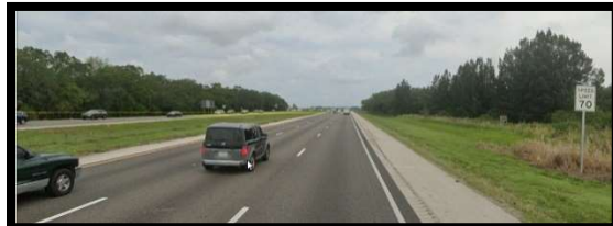
Begin Project MP 11.709 SLD 13075.000 Northbound, looking north
