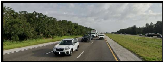
Begin Project MP 11.709 SLD 13075.000 Southbound, looking north
