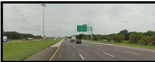
End Project MP 15.756 SLD 13075.000 Southbound, looking south
