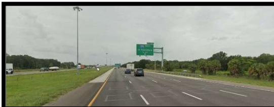
End Project MP 15.756 SLD 13075.000 Southbound, looking south
