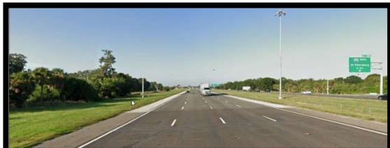
End Project MP 15.756 SLD 13075.000 Northbound, looking south
